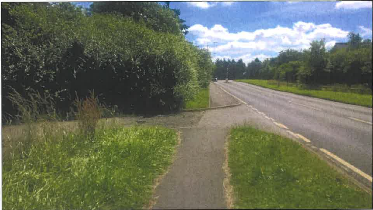
Figure 5: Crossing location at unnamed side road leading to a field
