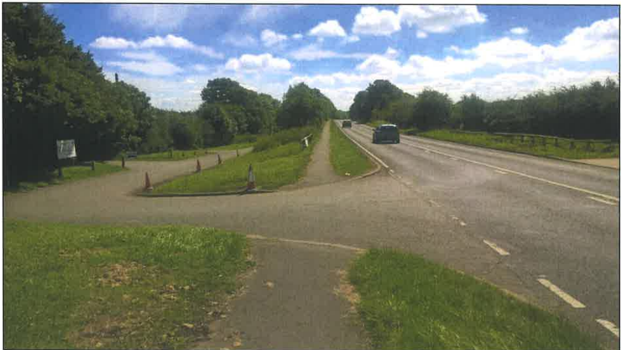
Figure 4: Crossing location at access road leading to Ajax Park
