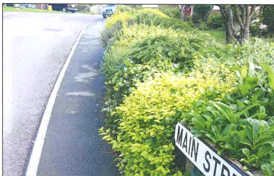
Figure 4 Minimum footway width of 1.1m on Main Street
