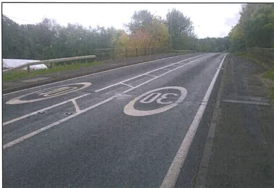
Figure 2 Footway on A423 Southam Road over Grand Union Canal Bridge
