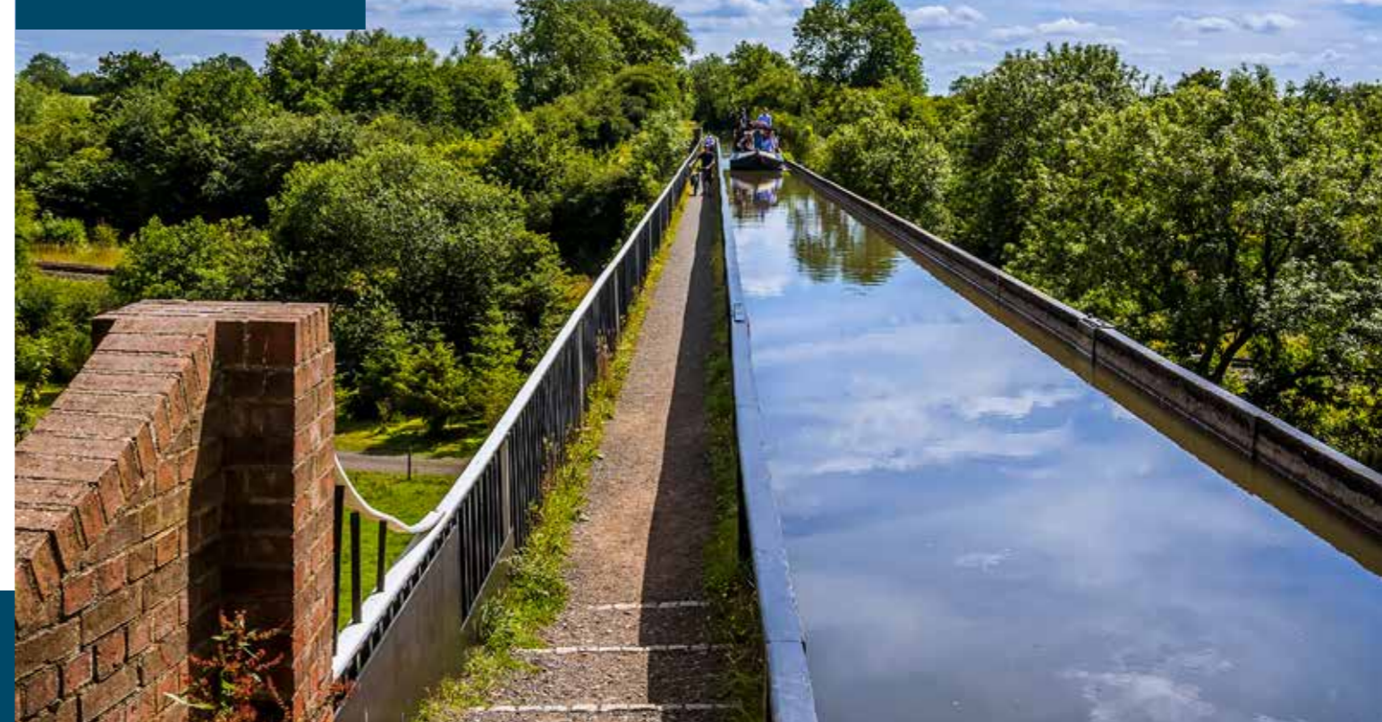
Photo from Shutterstock, Edstone Aqueduct
