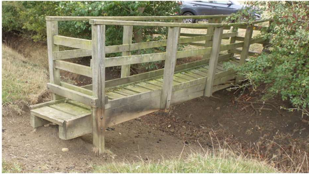
Tysoe – bridge replaced by volunteers
