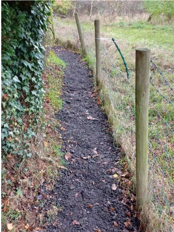
Stoned path – M173 Netherwood Lane
