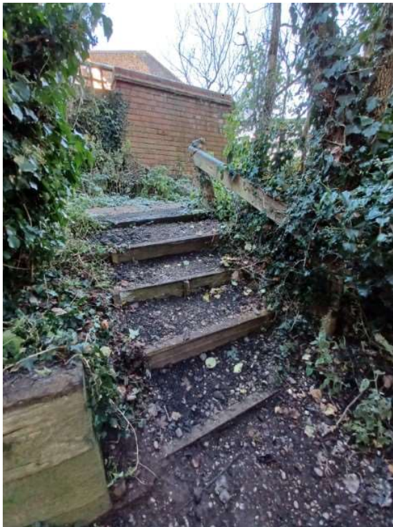
Step repairs M159 Long Brook Lane
