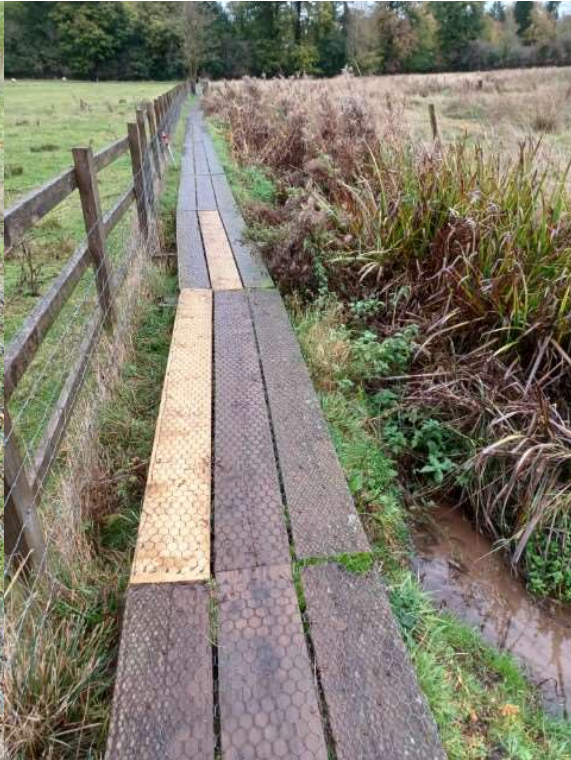
Boardwalk repairs – M192 Berkswell
