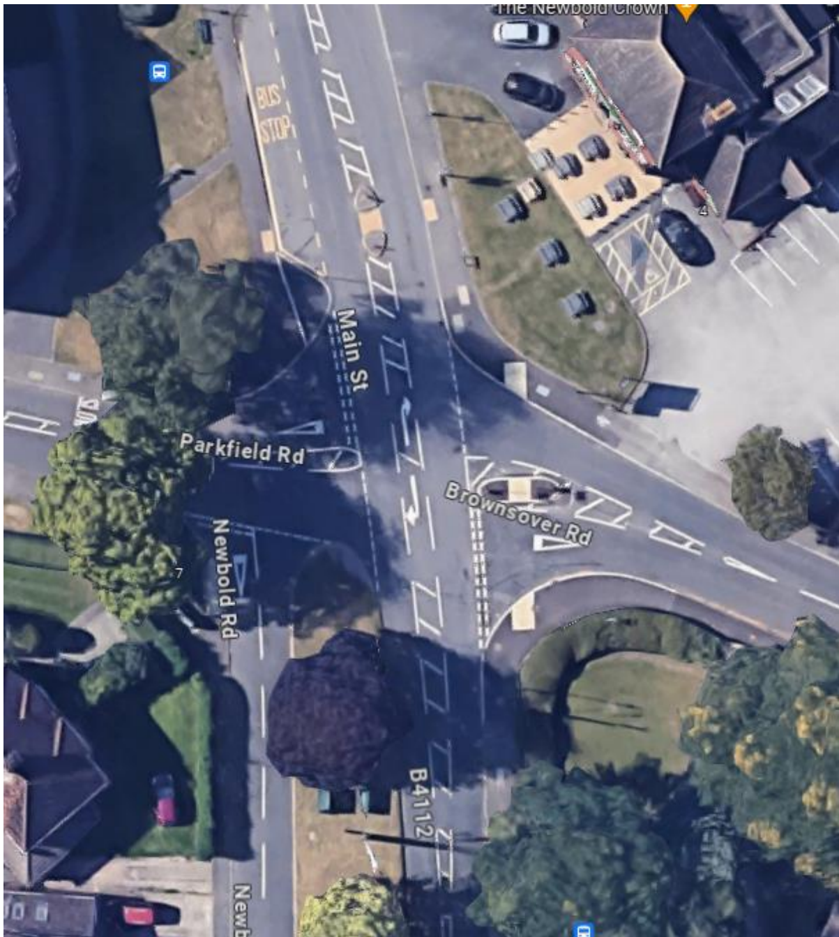
Overview image of the completed works.
