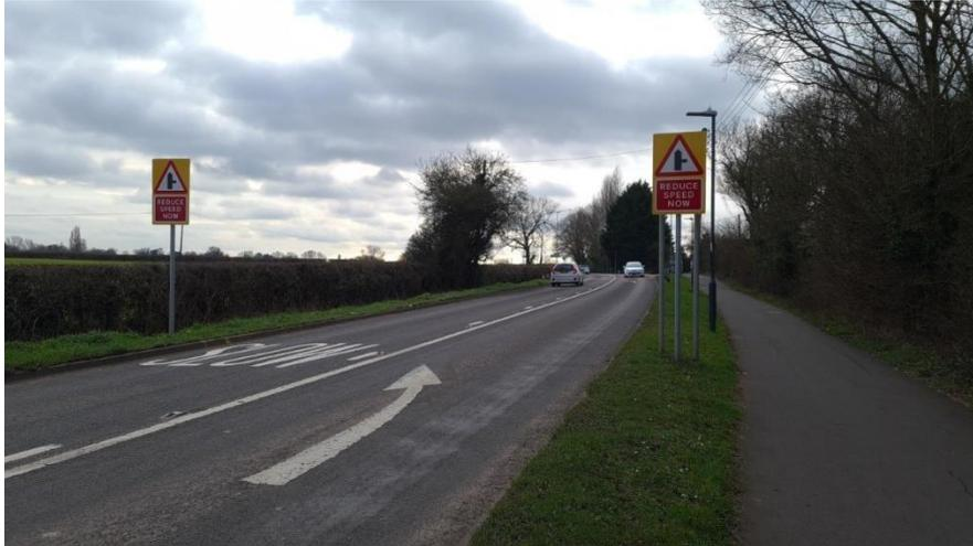
The works within the scheme gives the motorist an improved advance warning approaching the location. This has been achieved by installing two junction warning – reduce speed now signs, and “SLOW” road markings.
