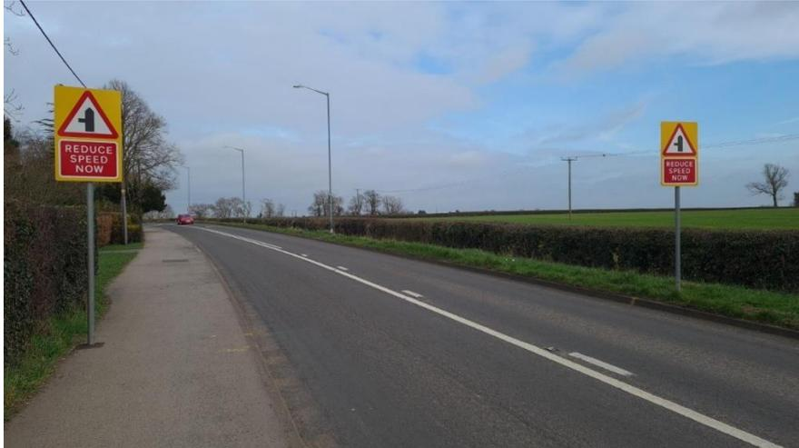
The works within the scheme gives the motorist an improved advance warning approaching the location. This has been achieved by installing two junction warning – reduce speed now signs, a further junction warning sign closer to the junction, and “SLOW” road markings.
