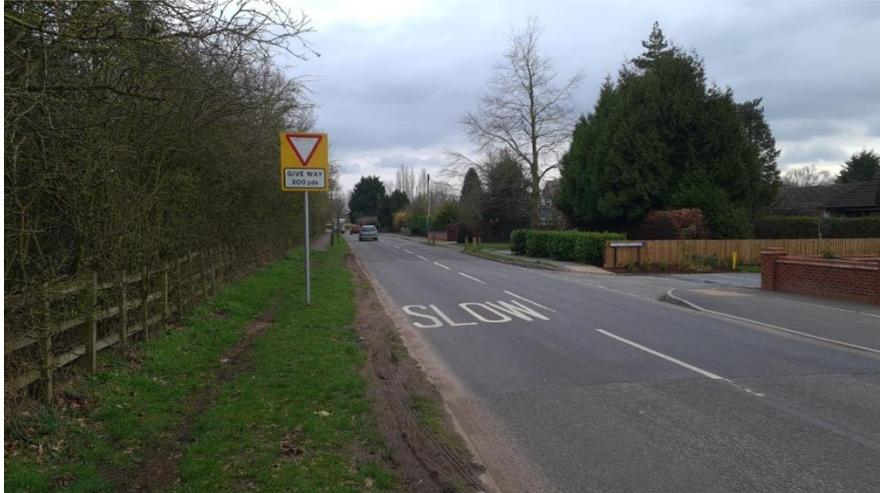
The works within the scheme gives motorists an improved advance warning approaching the location. This has been achieved by installing two junction warning – reduce speed now signs, and “SLOW” road markings. These have been installed at both 200 yards, and 100 yards.
