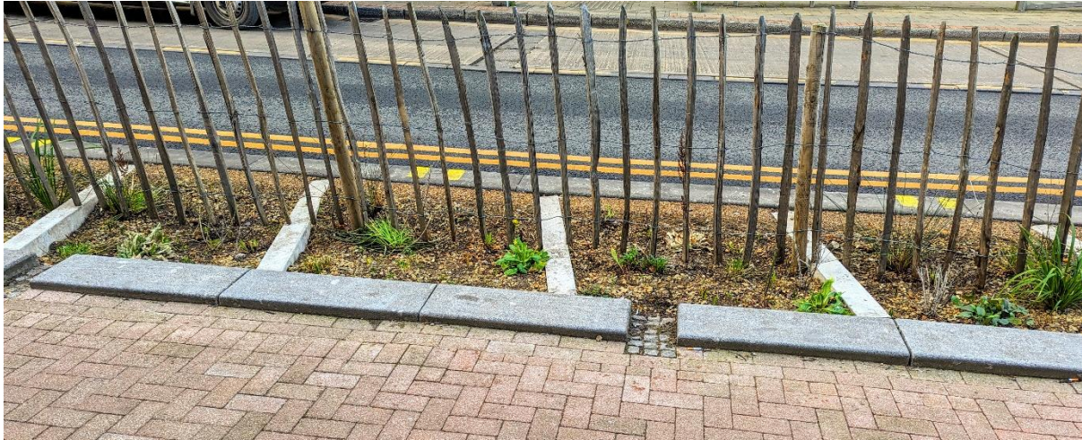
Figure 12 - Shallow swale / filter drain with check-dams (WCC 2023)
