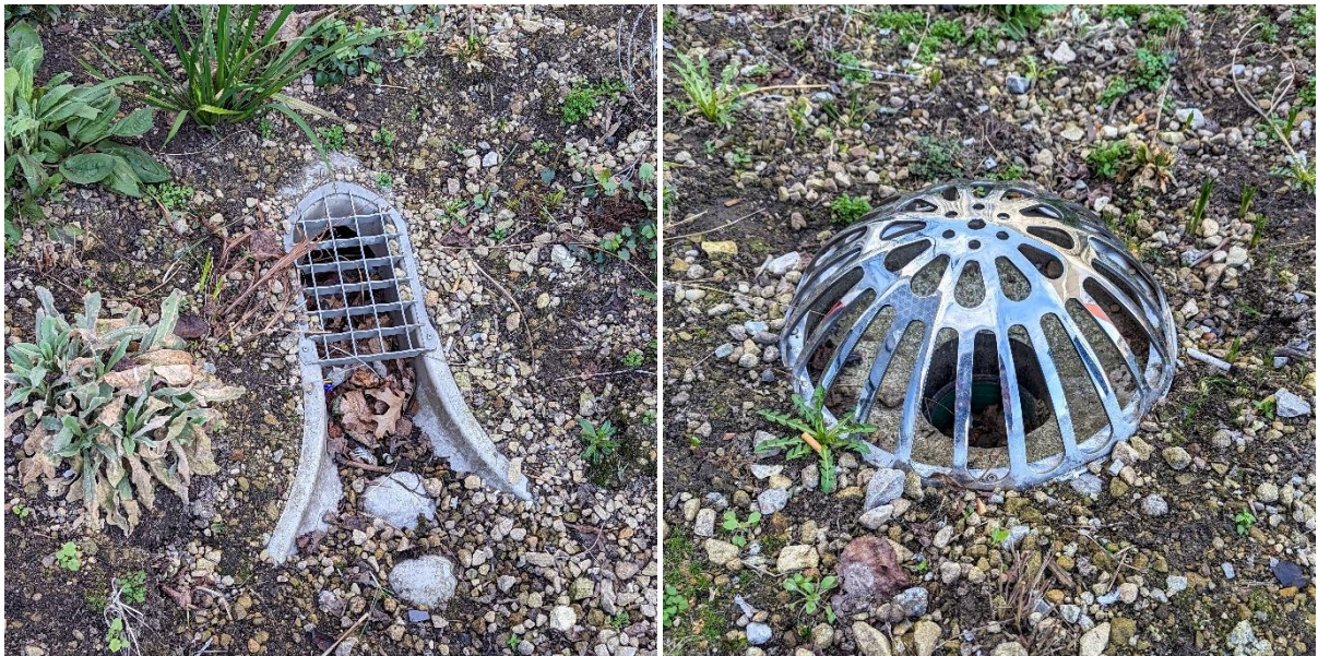
Figure 10 - Small scale inlet (left) and outlet (right) features (WCC, 2023)
