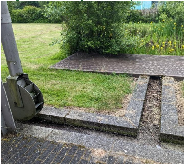
Figure 22 – Rill conveyance to small pond at back
