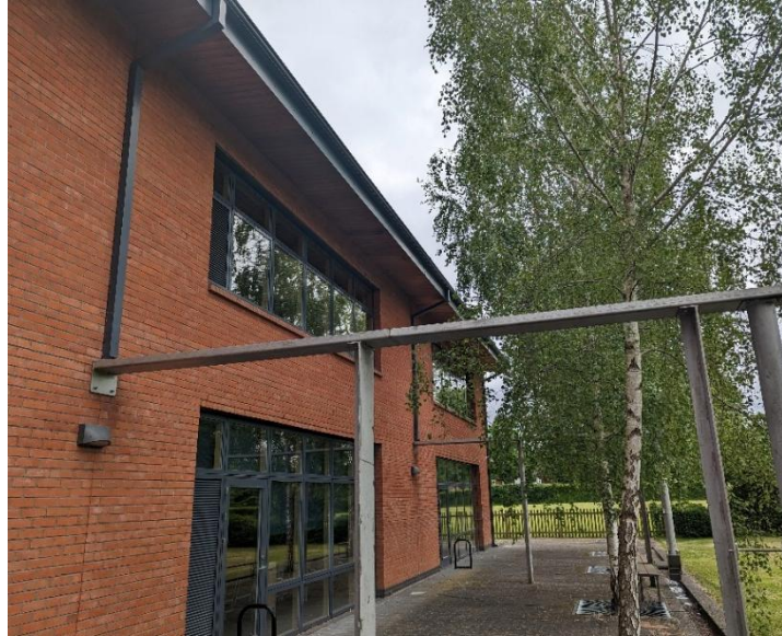
Figure 18 - Higher-level rainwater channel (long)
