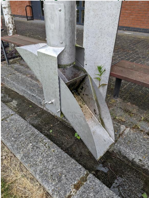
Figure 22 – Rill conveyance to small pond at back
