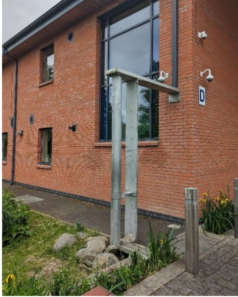
Figure 17 - Higher-level rainwater channel (short)
