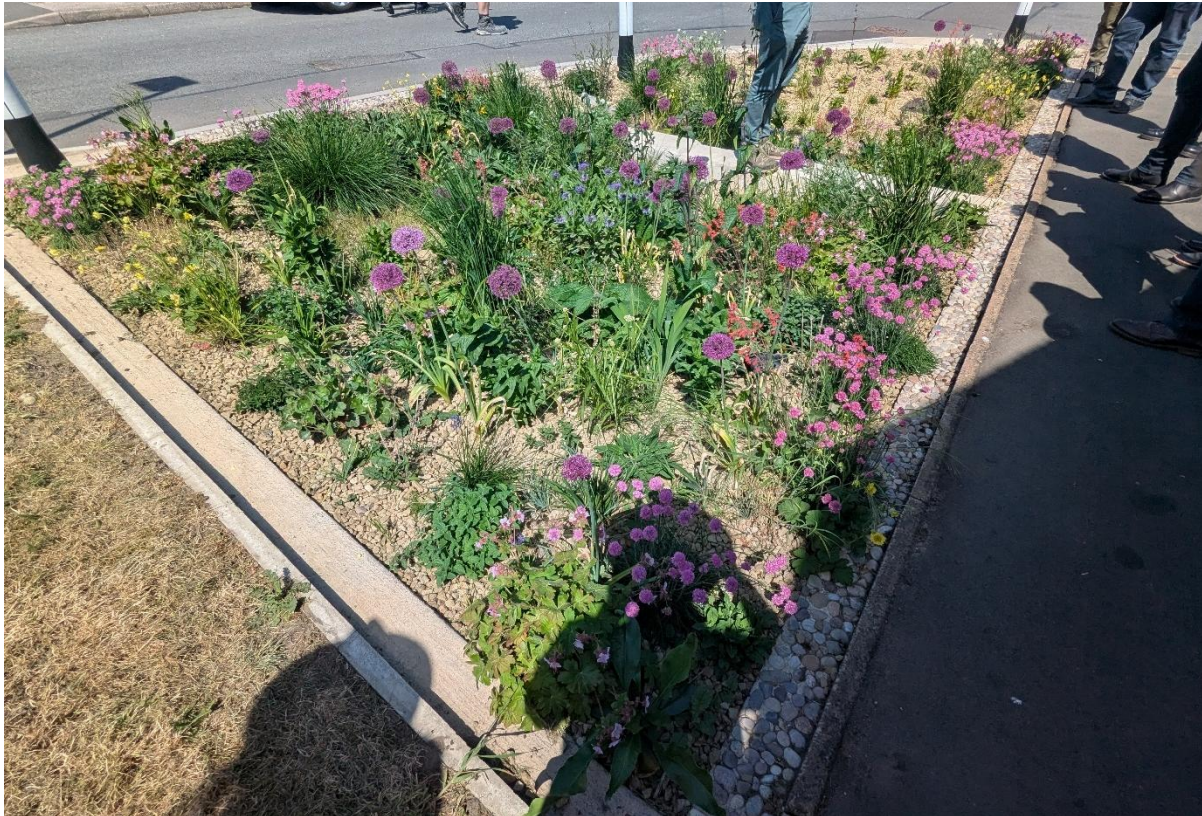
Figure 7 – Mansfield bio-retention / raingarden area (WCC, 2025)
