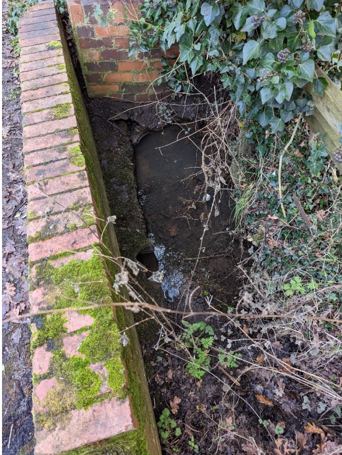
Figure 9 - 'Plank Lane East Culvert' upstream inlet
