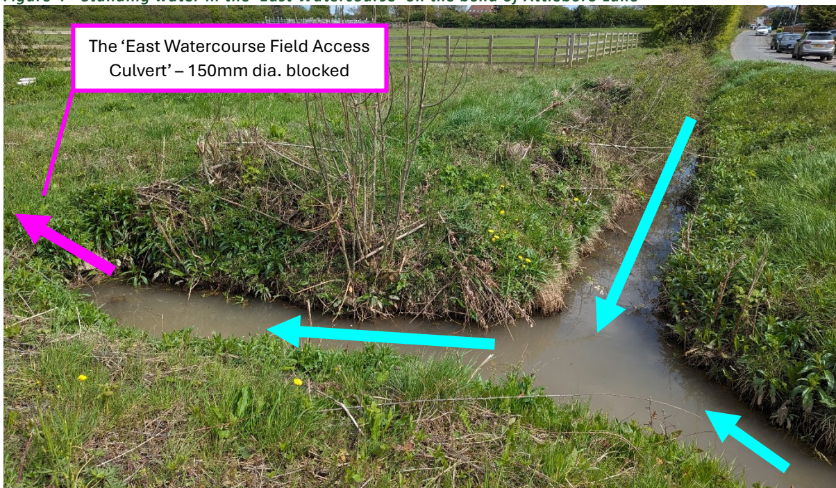
Figure 4 - Standing water in the 'East Watercourse' on the bend of Attleboro Lane
