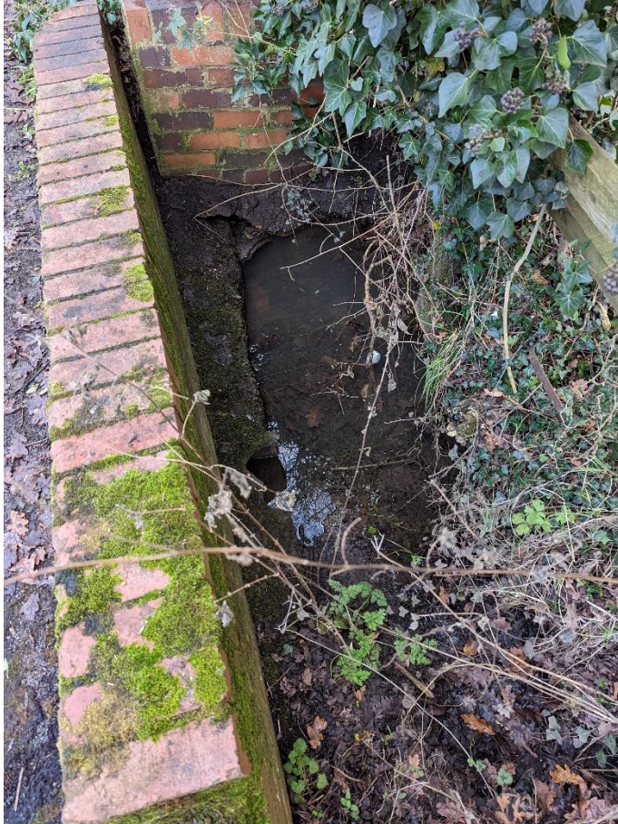
Figure 9 - 'Plank Lane East Culvert' upstream inlet
