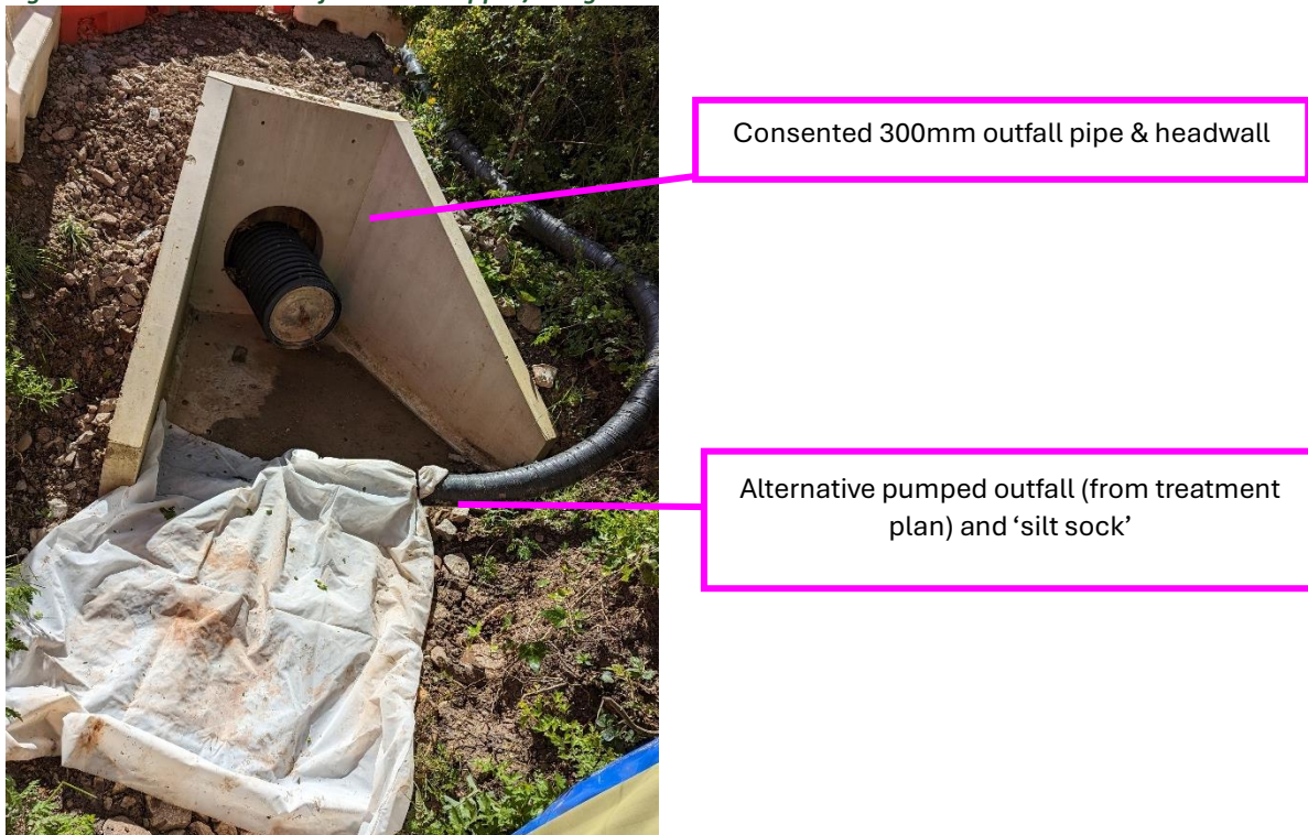
Figure 5 - Pond 165.2 Outfall with stopper/bung
