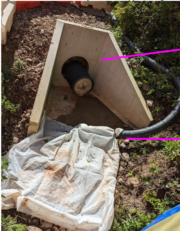
Figure 5 - Pond 165.2 Outfall with stopper/bung
