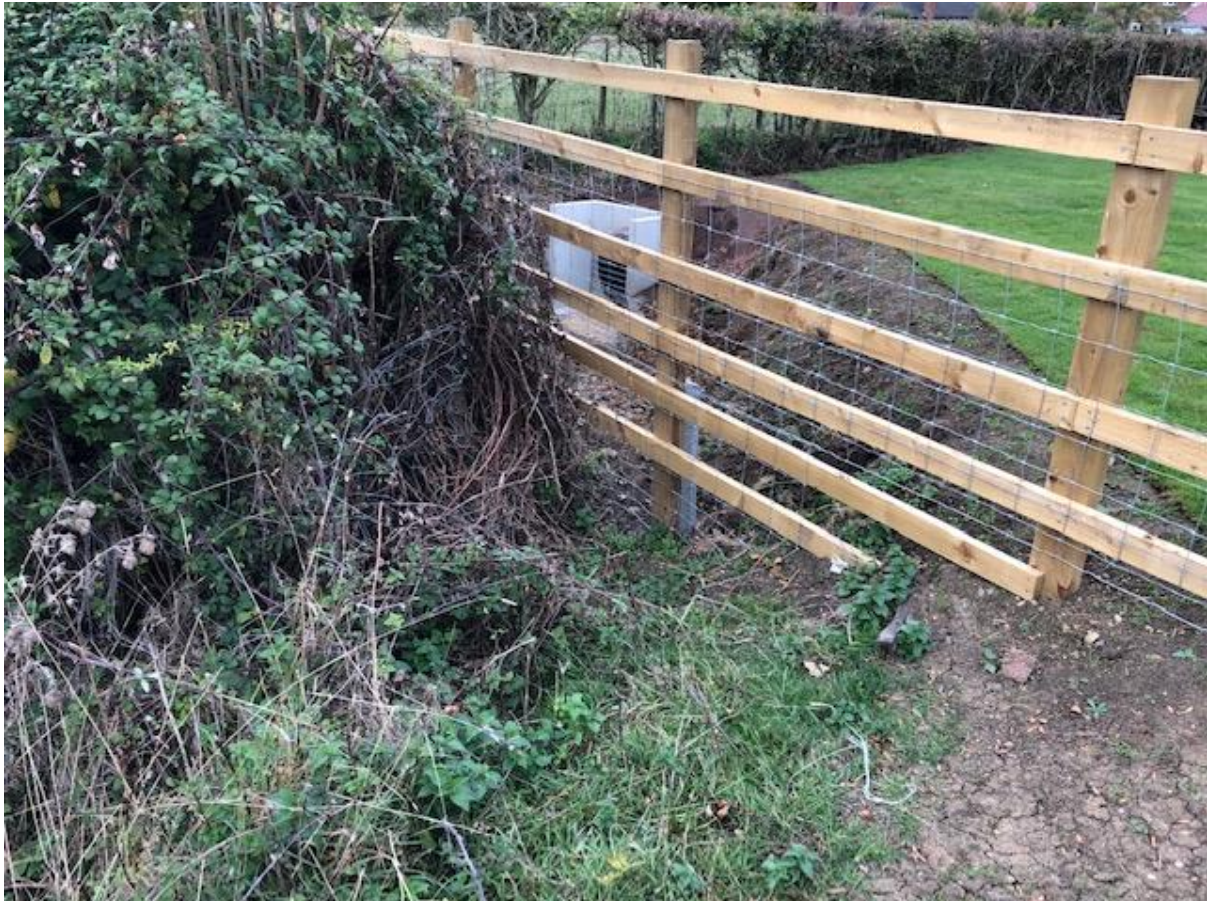
Figure 19 - A fence through a watercourse (unconsented and not acceptable; WCC 2018)
