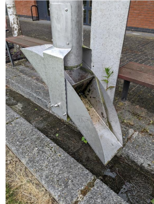
Figure 5 - Tipping bucket rainwater pipe outfall
