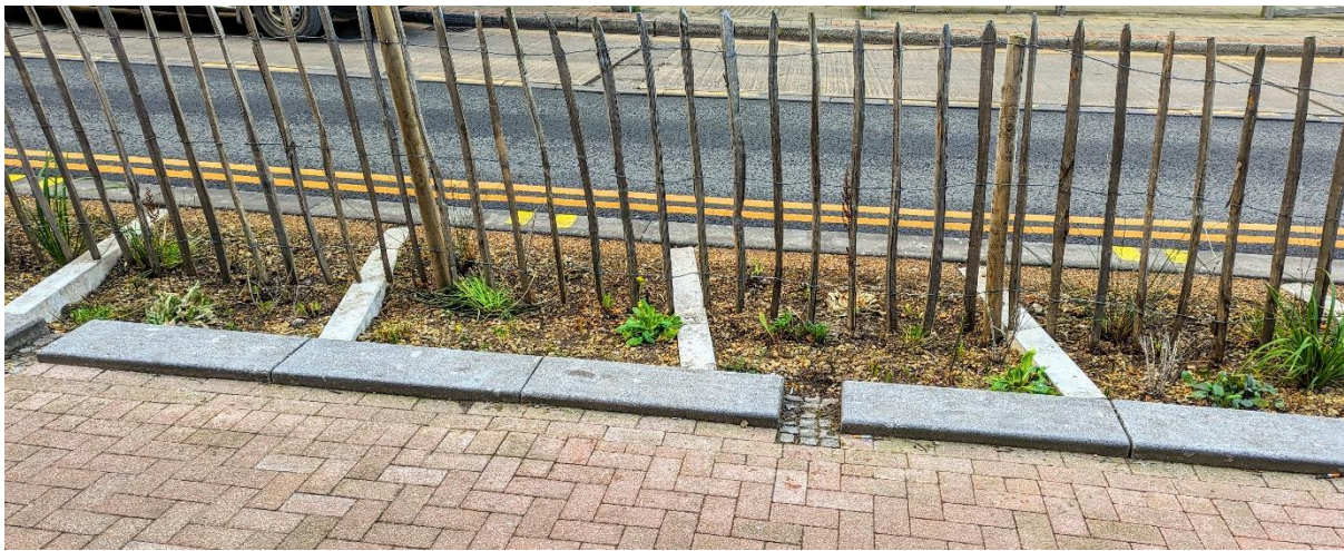
Figure 14 - Shallow swale / filter drain with check-dams
