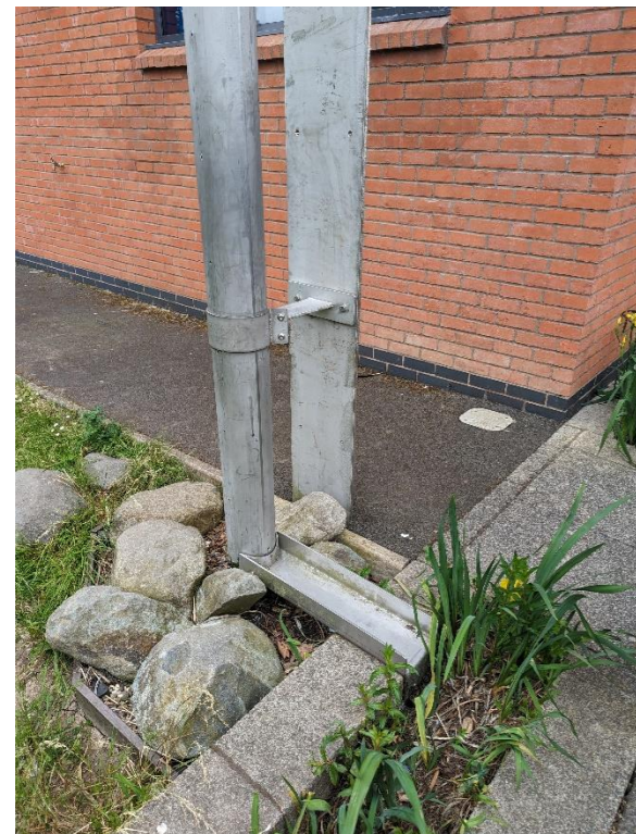
Figure 3 (left) - Rainwater pipe with small orifices
