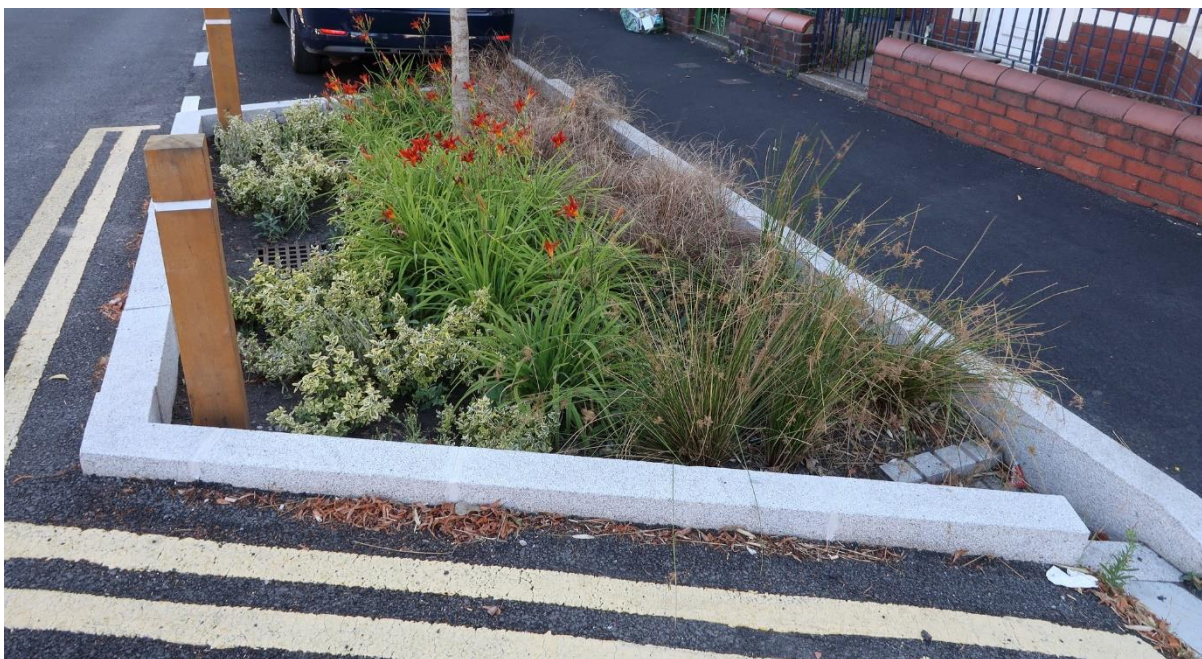
Figure 11 - Greener Grangetown bio-retention/raingarden area 6
