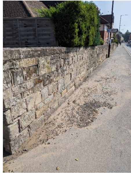
Figure 3 – site photos taken the day after the flood event showing evidence of a flow path from Priory Park issuing on to the highway.
