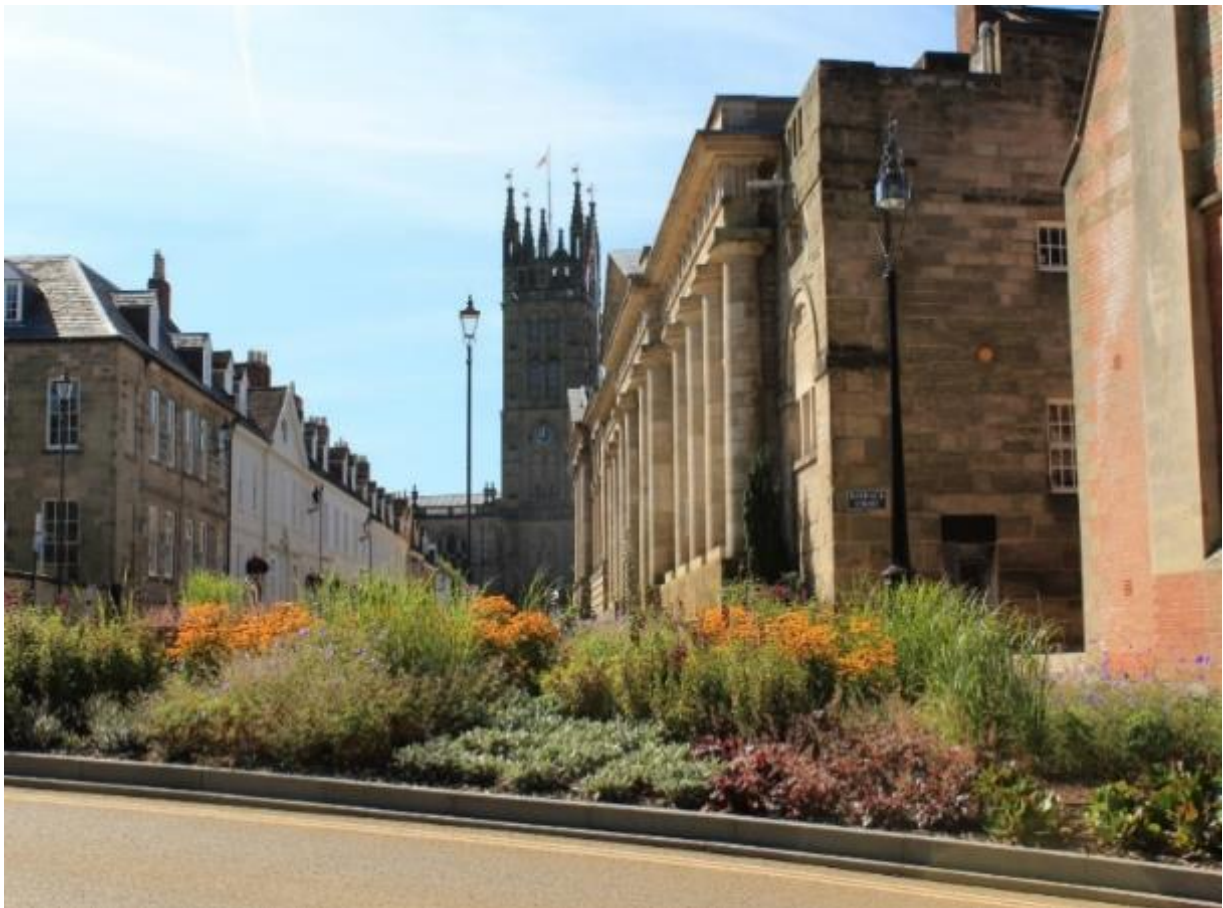
Urban greening and SuDS, Warwick town centre
