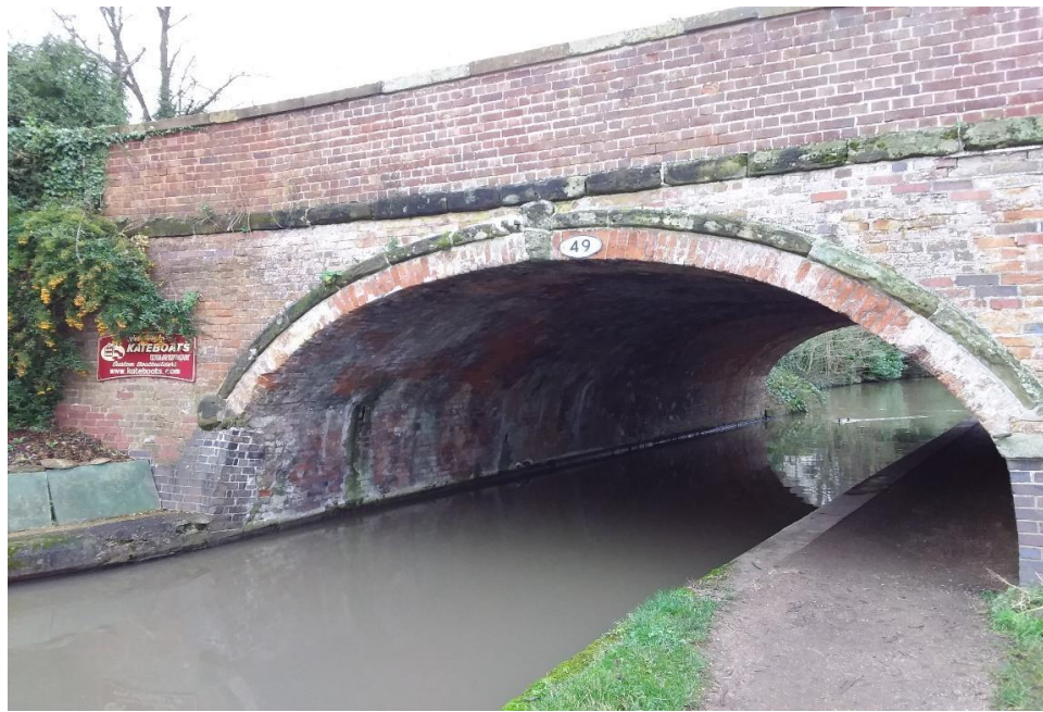
Structure B – A429 road bridge crossing the Grand Union Canal, as seen from the east
