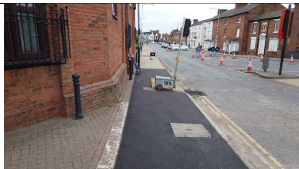
Works completed at Clopton Road
