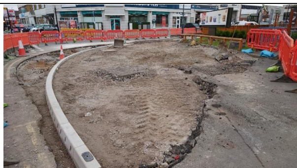
Western Road footway works
