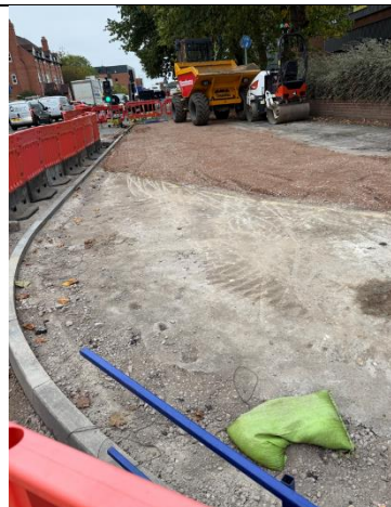
Kerbs have been installed at Wharf Road
