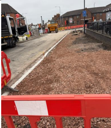
Excavation works at Arden Street
