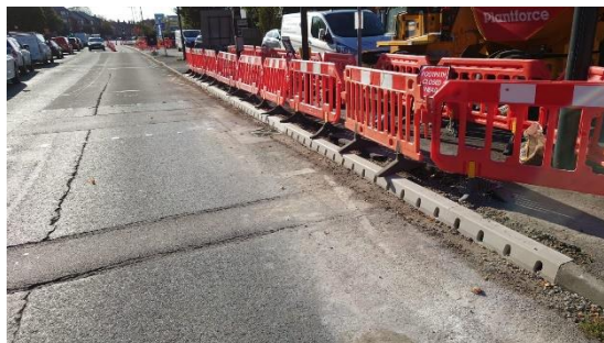
Kerbs have been installed at the Park Road roundabout.
