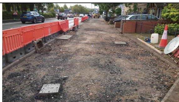
Footway excavation works outside Maybird Roundabout.
