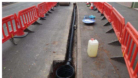
Drainage pipes being installed.
