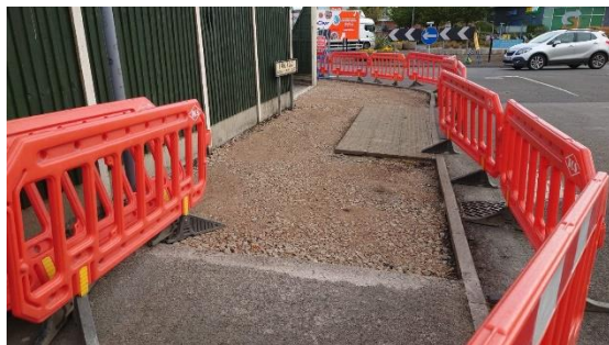
Tactiles installed and footway prepped for footway resurfacing works.
