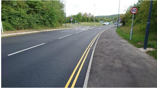
Carriageway resurfacing from Bishopstone roundabout to St Peters Way Junction.
