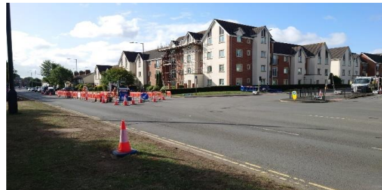
Site activities carried out adjacent to Hamlet Way.
