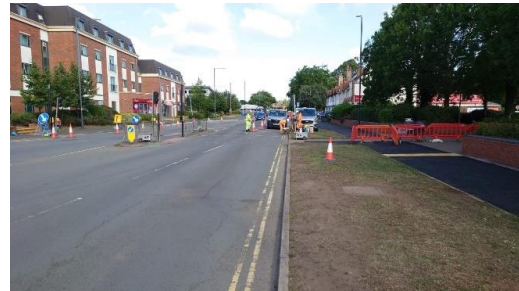
Temporary traffic signals installed at Hamlet Way.
