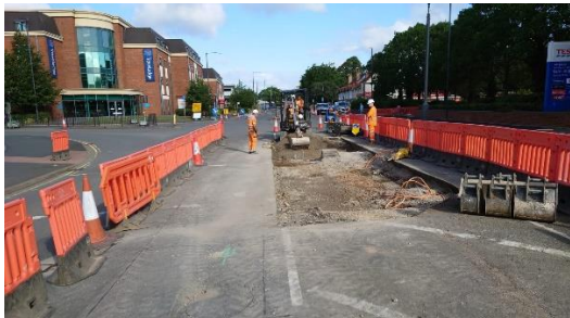
Carriageway excavation works outside Tesco.
