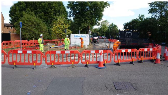
Excavating to install new traffic signals at Josephs Way.
