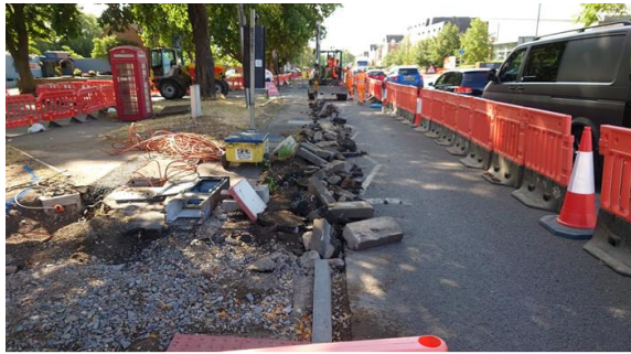
Excavation works taking place by Justin's Avenue.
