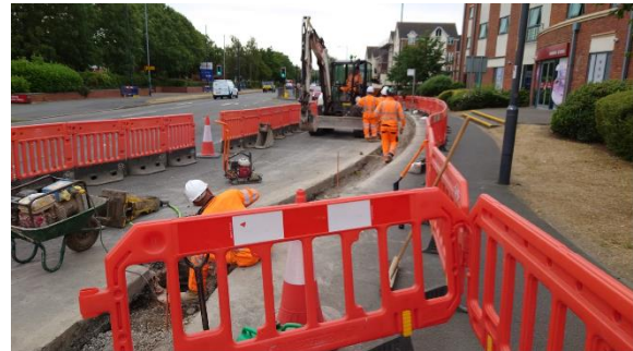
Kerbs being installed by Hamlet Way.
