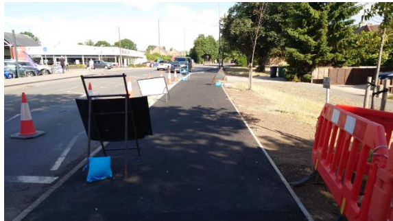
Works completed on Oakleigh Road.
