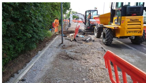
Kerb edgings being installed.
