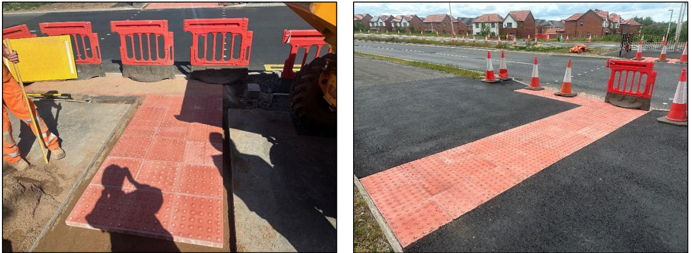
Figure 2 Phase G – Tactile Paving Installation
