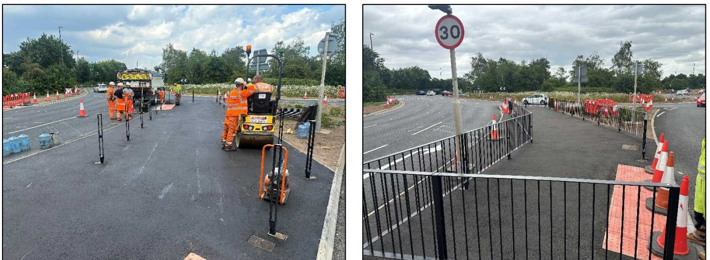
Figure 3 Phase G – Tarmac Surfacing & Guardrail Installation
