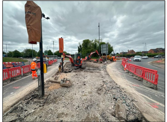
Figure 7 Phase L – Splitter Island Kerb Removal & Excavation
