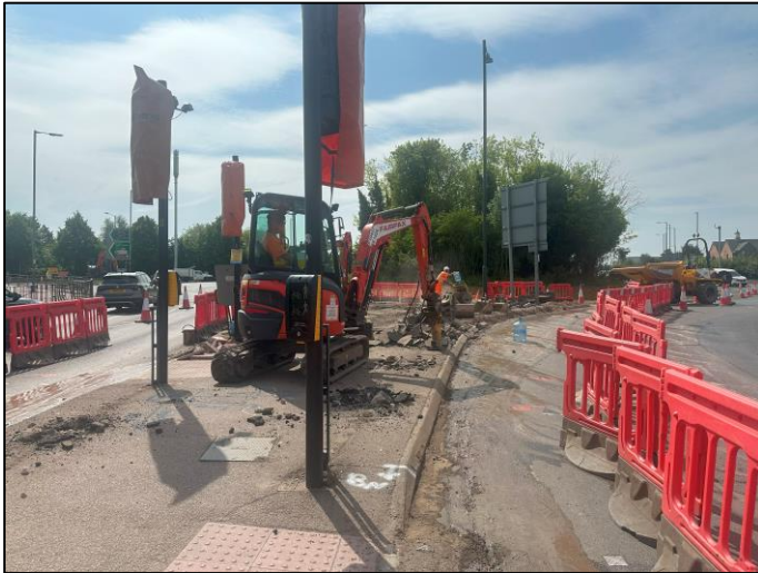
Figure 7 Phase L – Splitter Island Kerb Removal & Excavation
