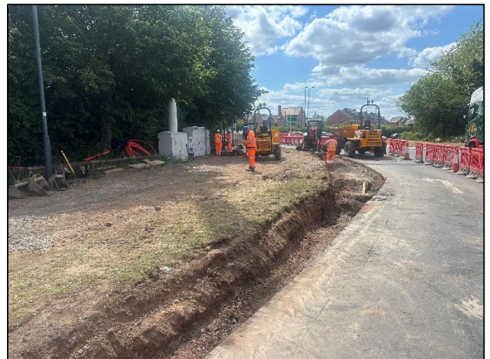
Figure 11 Phase M – Existing Kerb Removal & Road Box Excavation
