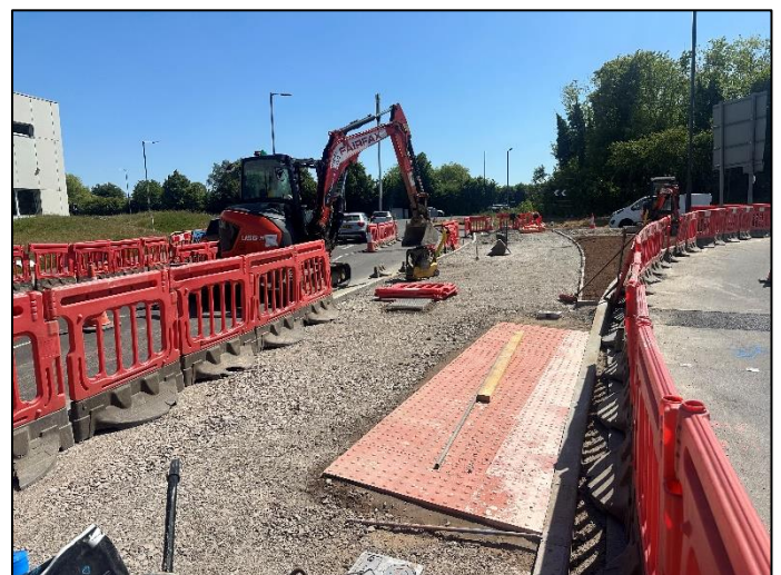
Figure 8 Phase L - Splitter Island New Kerb Alignment & Tactile Installation
