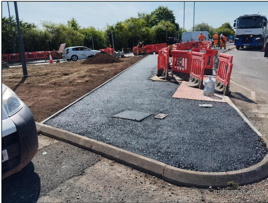
Figure 1 Phase K – Splitter Island Binder Course
