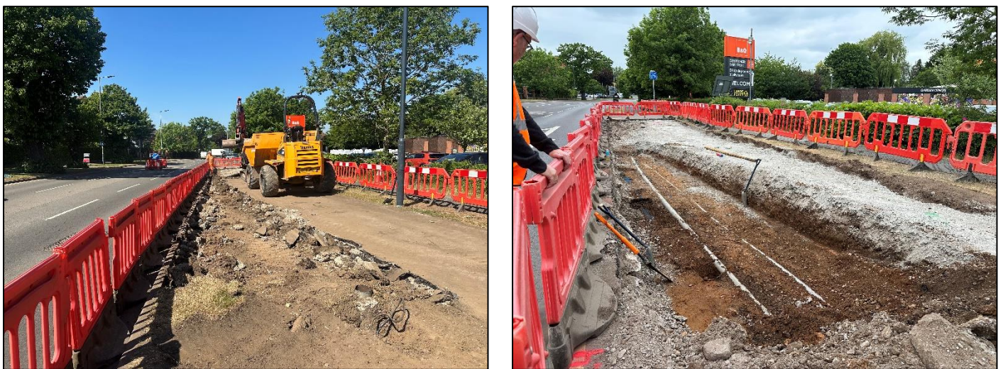
Figure 9 Phase J – Verge Excavation & Utility Protection
