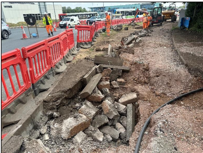
Figure 11 Phase M – Existing Kerb Removal & Road Box Excavation
