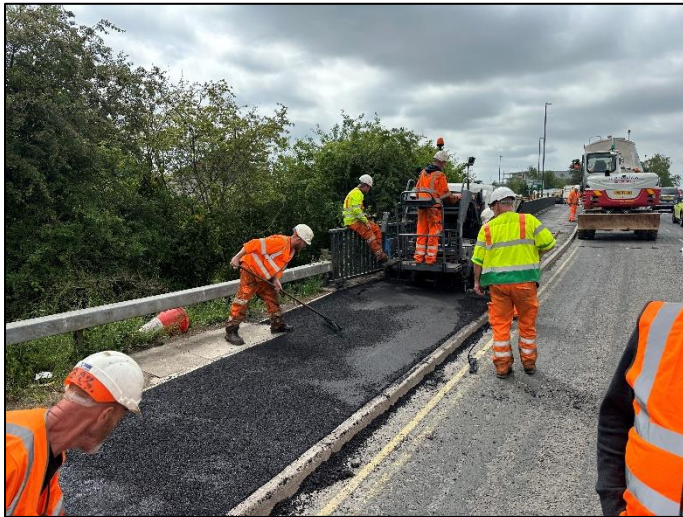
Figure 4 Phase F – Upper Footpath Surfacing
