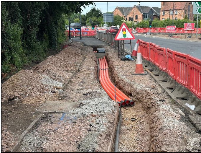
Figure 10 Phase M – Traffic Signal Ducting Installation
