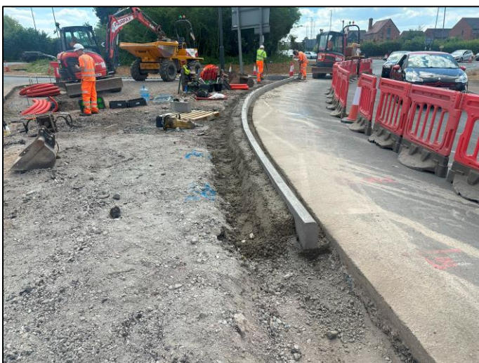
Figure 8 Phase L - Splitter Island New Kerb Alignment & Tactile Installation
