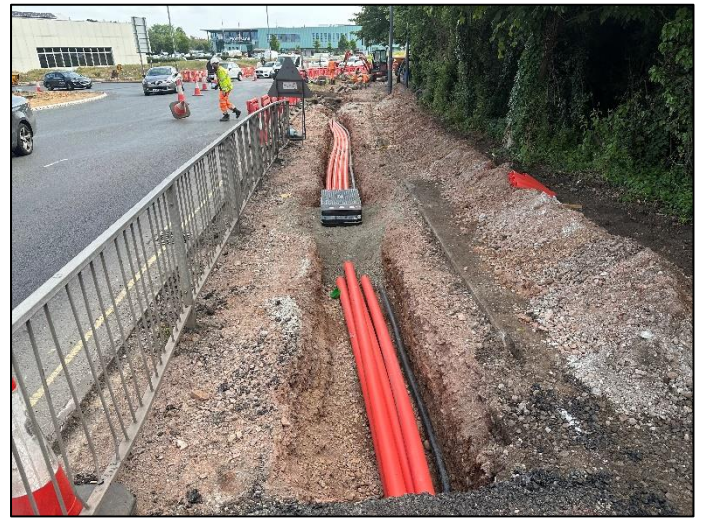
Figure 10 Phase M – Traffic Signal Ducting Installation
