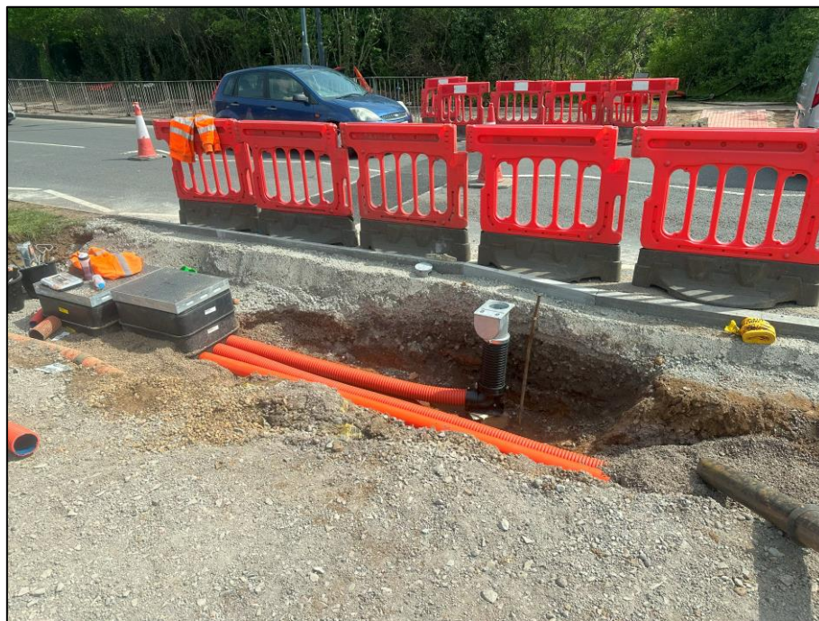
Figure 1 Phase K – Traffic Signal Cable Ducting Installation
