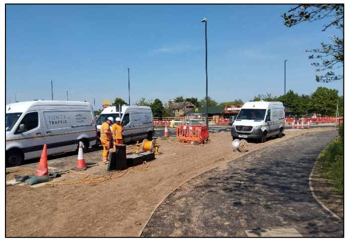
Figure 6 Phase B – New Pedestrian Crossing Tactile and Traffic Signal Cable Installation
