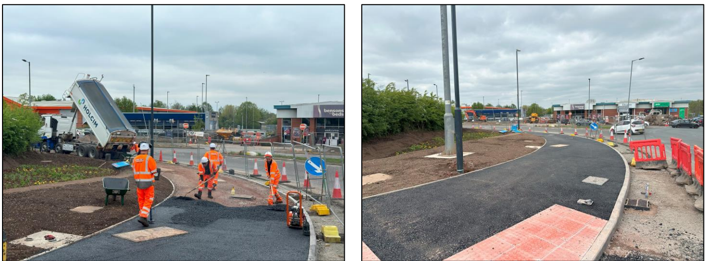
Figure 5 Phase H - Footway surfacing and Tactile Paving
