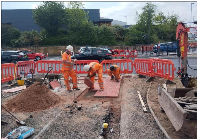
Figure 6 Phase B – New Pedestrian Crossing Tactile and Traffic Signal Cable Installation
