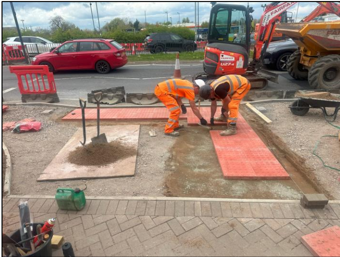
Figure 2 Phase K - Tactile Paving Installation Completed
