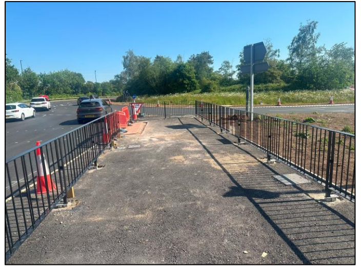
Figure 4 Phase J – Pedestrian Guard Rail Installation
