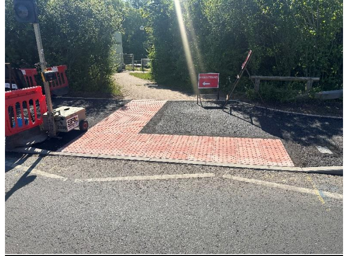
Figure 2 Phase K - Tactile Paving Installation Completed
