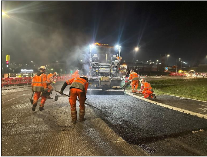
Figure 3 - Tarmac Surfacing
