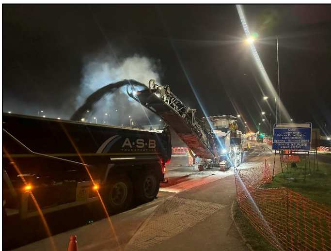
Figure 2 Planing Existing Road Surface
