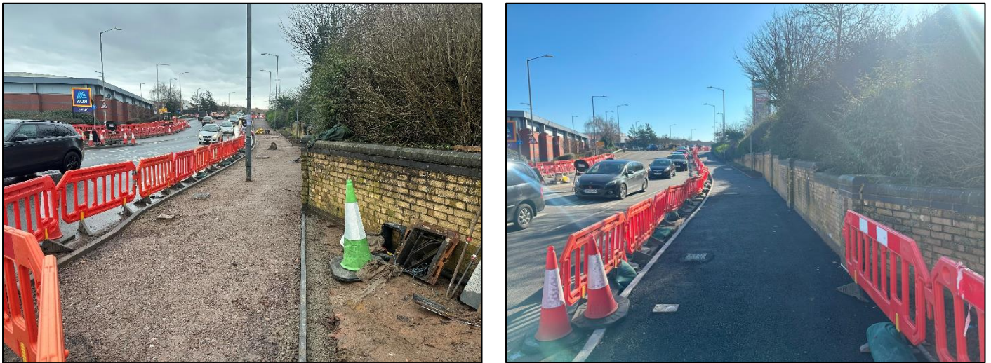
Figure 3 Phase D - New Footpath Construction Before and After Binder Layer
