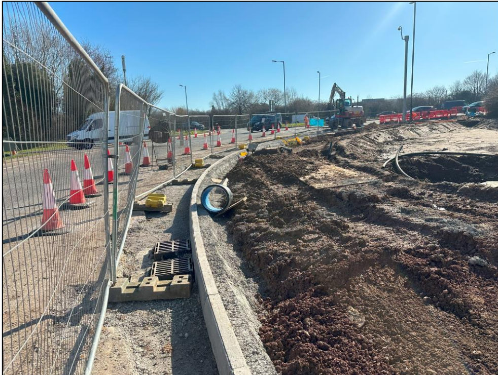
Figure 4 Phase H - New Kerb Alignment and Attenuation Pond
