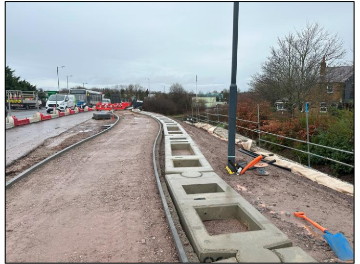
Figure 2 Phase F - Smarcraft VRS foundation installation
