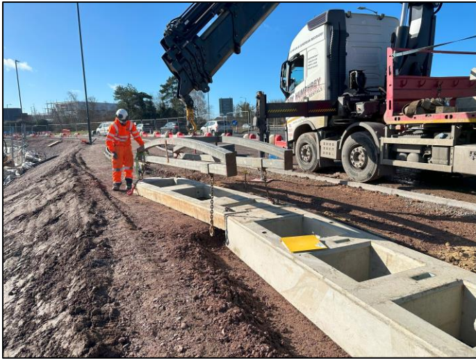
Figure 2 Phase F - Smarcraft VRS foundation installation
