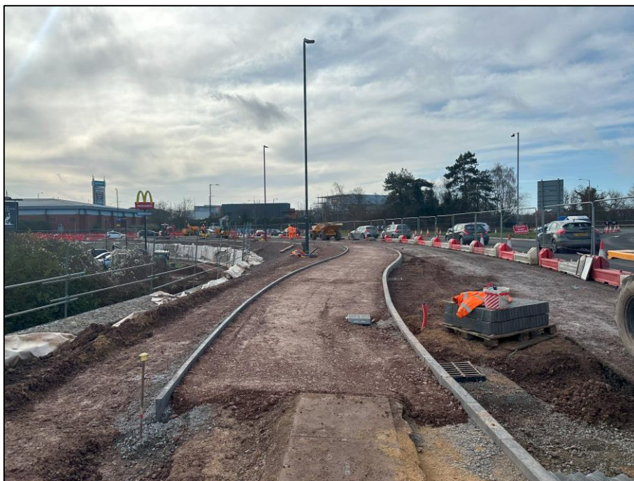
Figure 1 Phase F – Kerb and Edging Installation
