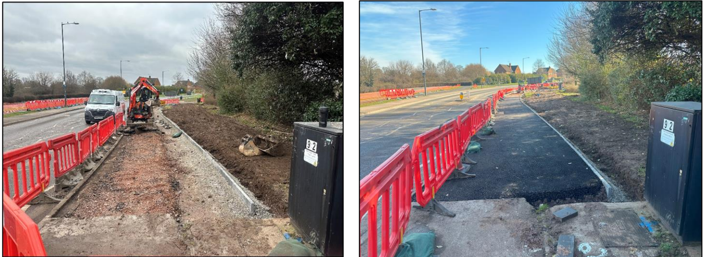
Figure 5 Phase B – Footway Binder Course
