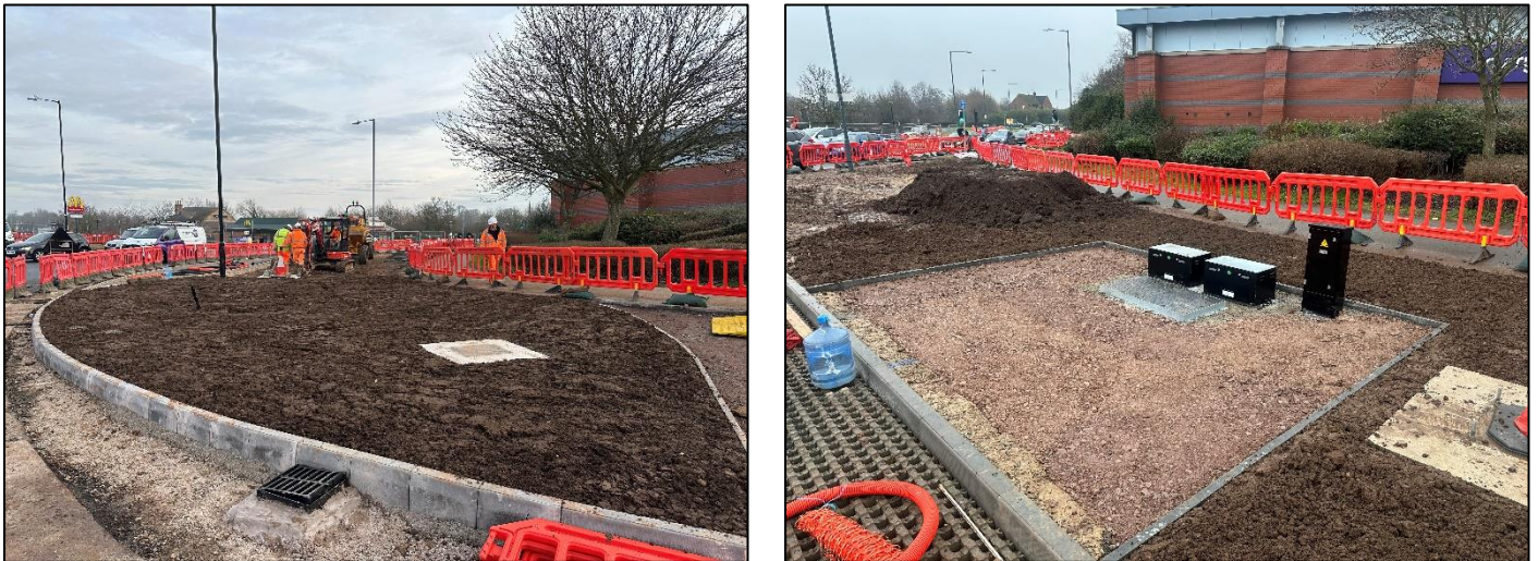
Figure 5 Phase B - Traffic Signal Maintenance Bay Construction
