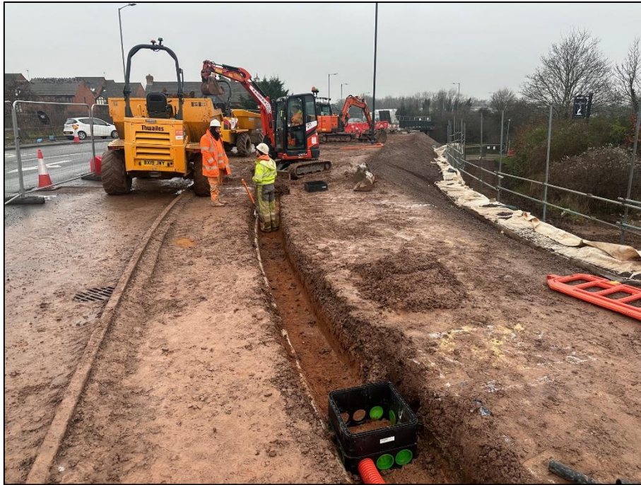
Figure 2 Phase F - Street Lighting Trench and Ducting Installation
