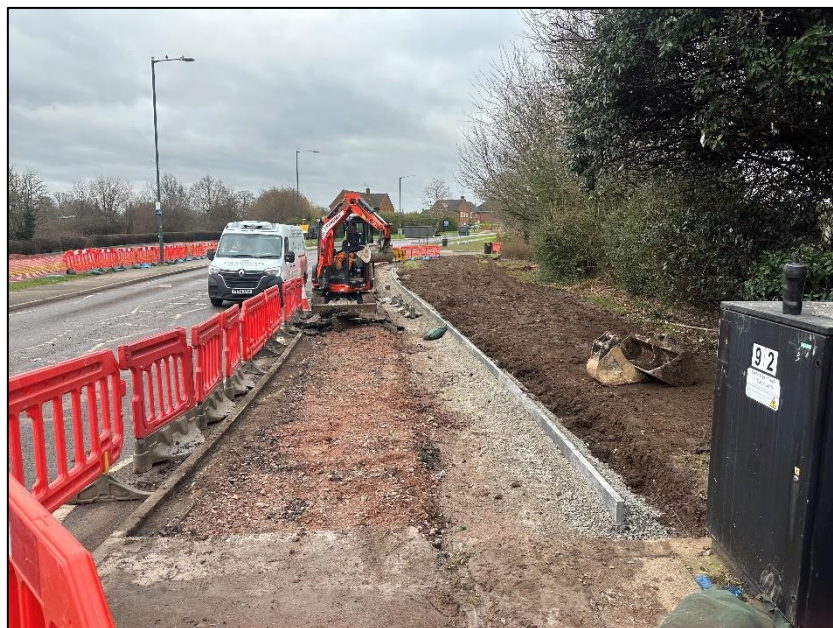
Figure 6 Phase B – Widened Footway Works
