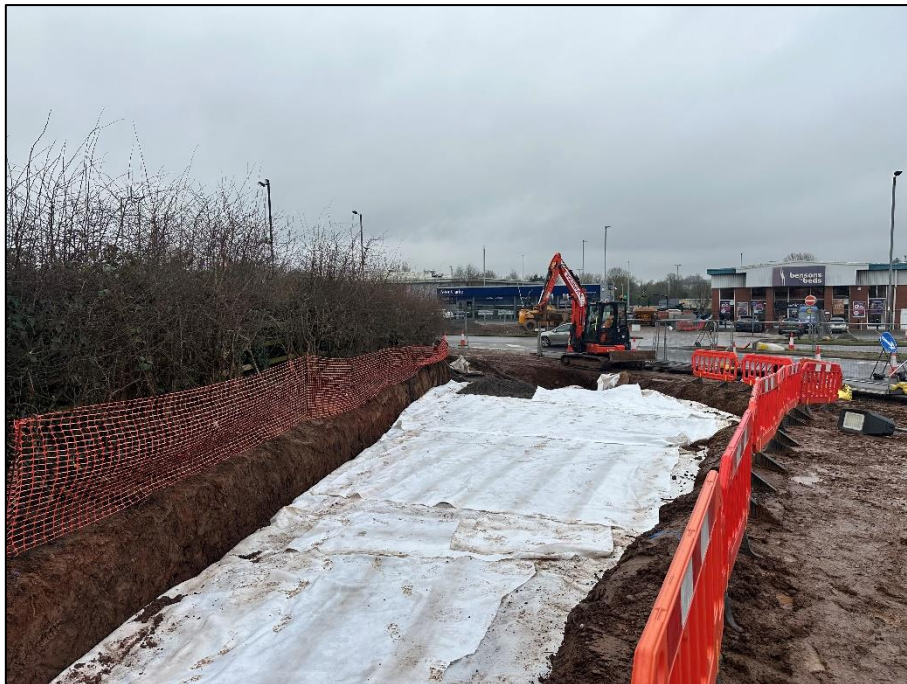
Figure 4 Phase H - Highway Drainage Attenuation Basin
