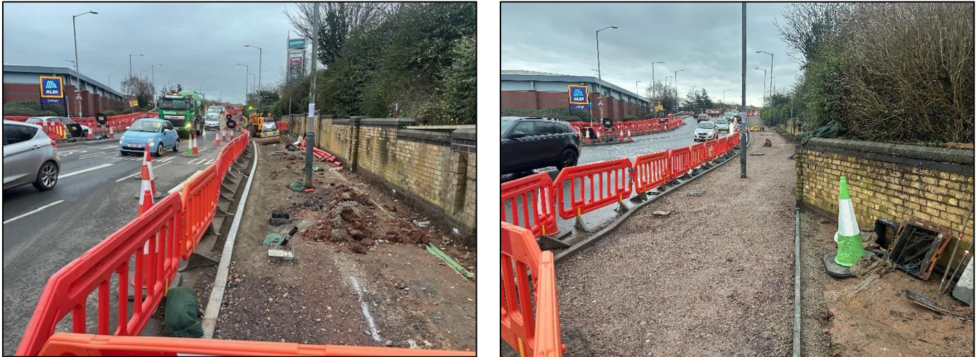
Figure 3 Phase D - New Footpath Construction
