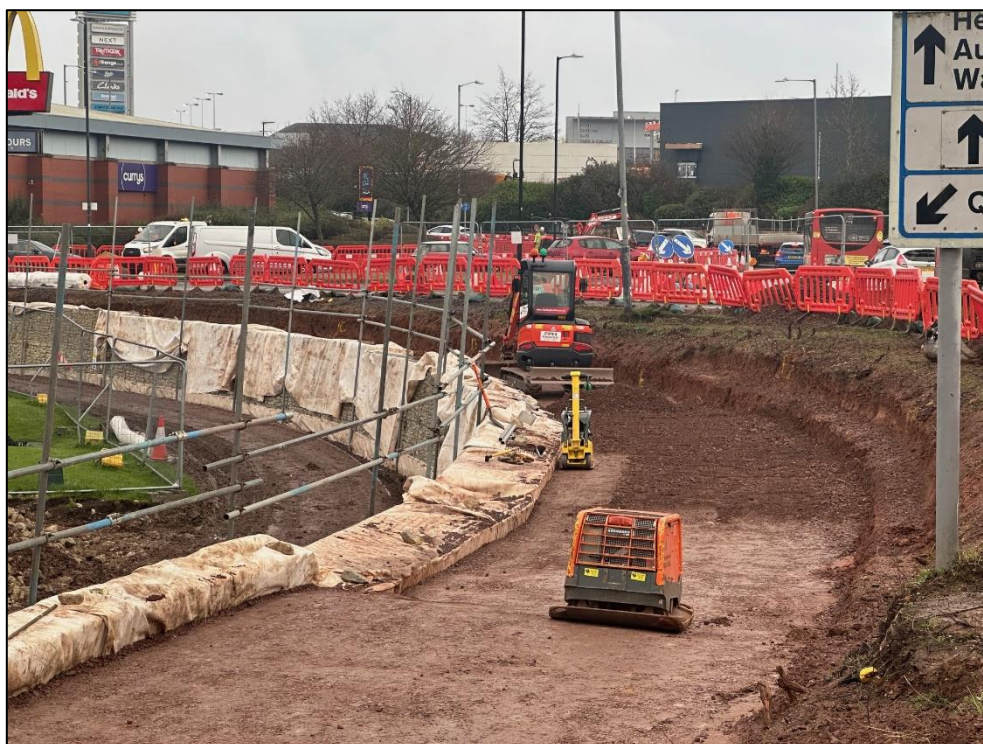
Figure 1 Gabion Retaining Wall Backfill Works
