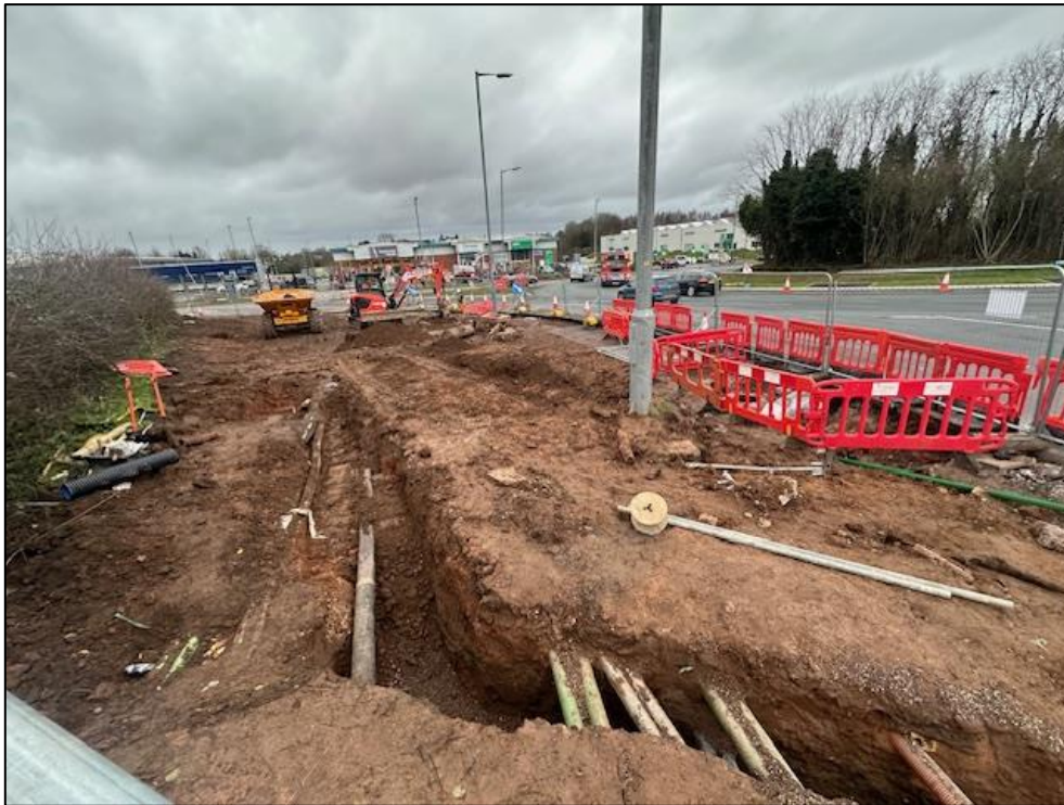
Figure 4 Phase H Drainage Duct Construction and Service Diversions
