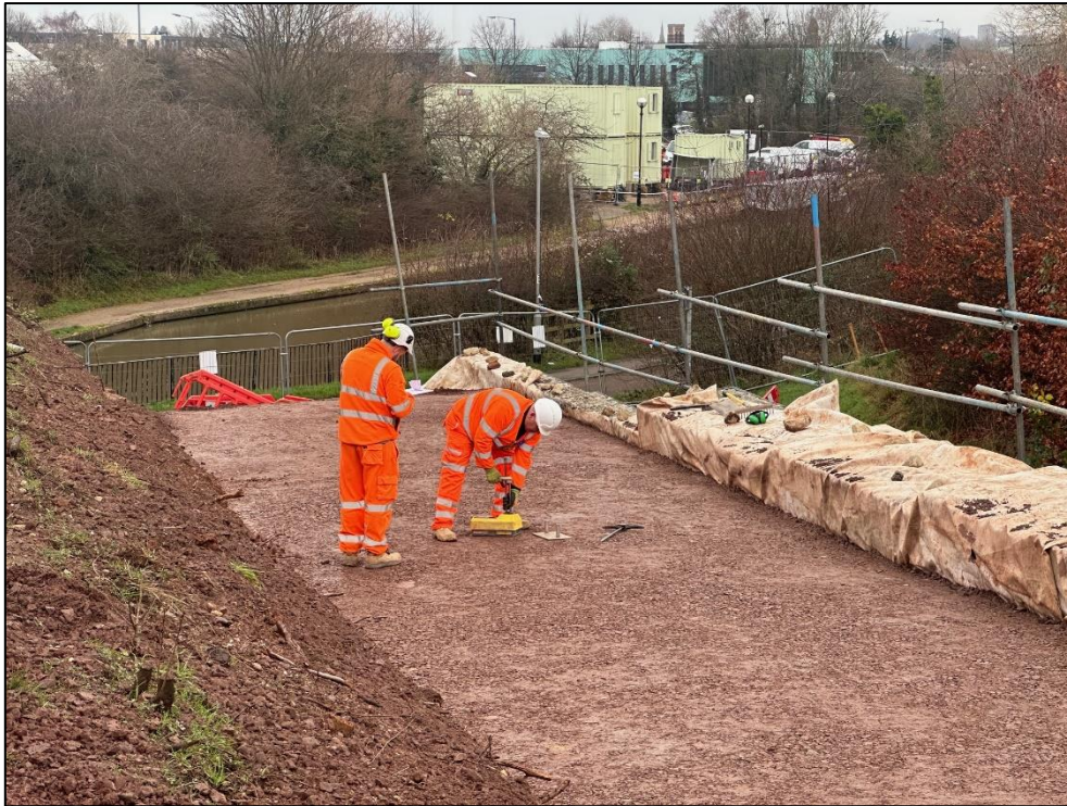
Figure 2 Gabion Retaining Wall Backfill Density Testing
