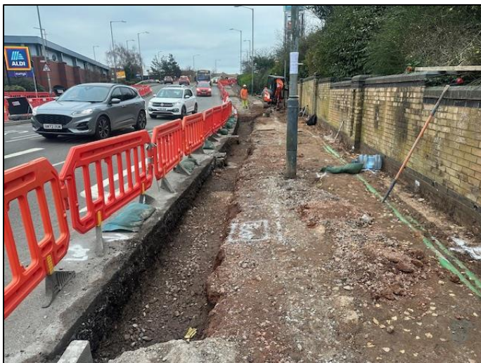
Figure 3 Phase D New Kerb-line Construction
