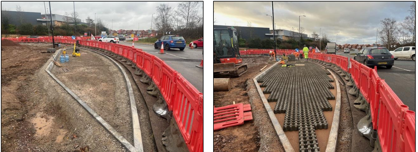
Figure 5 Phase B Traffic Signal Maintenance Bay Construction
