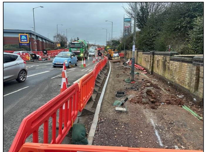
Figure 3 Phase D New Kerb-line Construction
