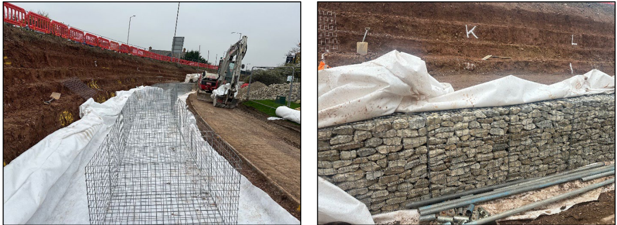
Figure 1 - Gabion Basket Construction and Facing
