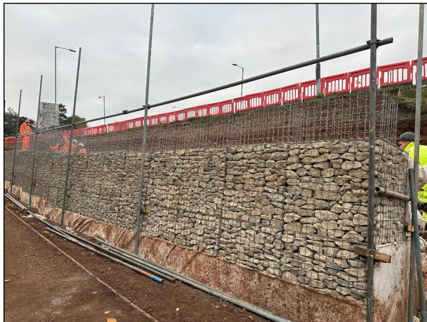
Figure 2 - Gabion Retaining wall 3m height
