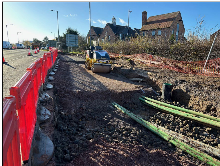
Figure 4 Phase H - Widened Lane Construction
