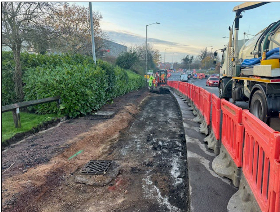
Figure 3 Phase D - Excavation of Existing Footpath
