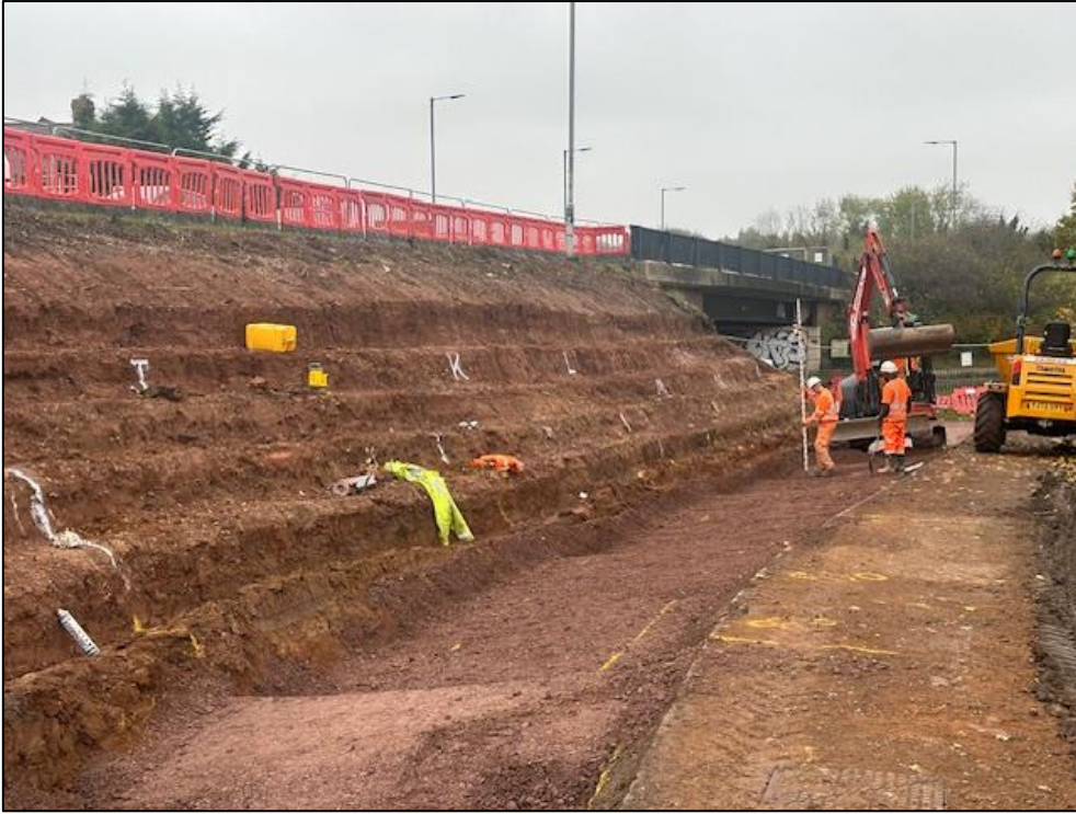
Figure 2 Gabion Base Formation
