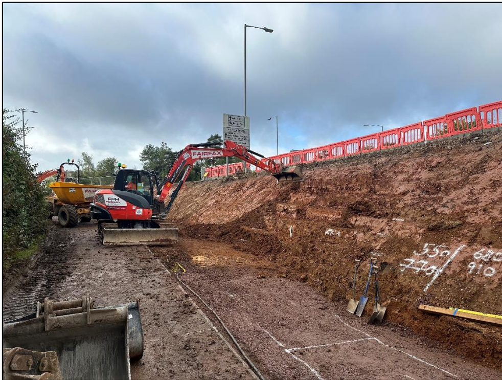
Figure 1 Embankment Stepping Works
