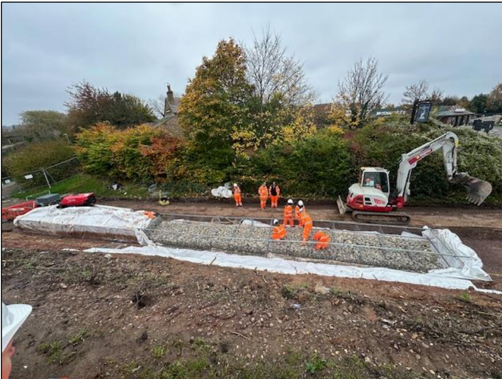
Figure 3 Gabion Basket Construction
