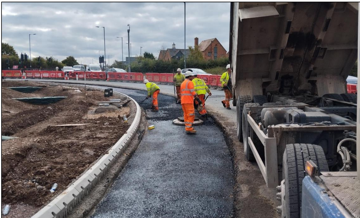
Figure 3 Old Warwick Road Roundabout – Laying of The Upper Structural Road Layers
