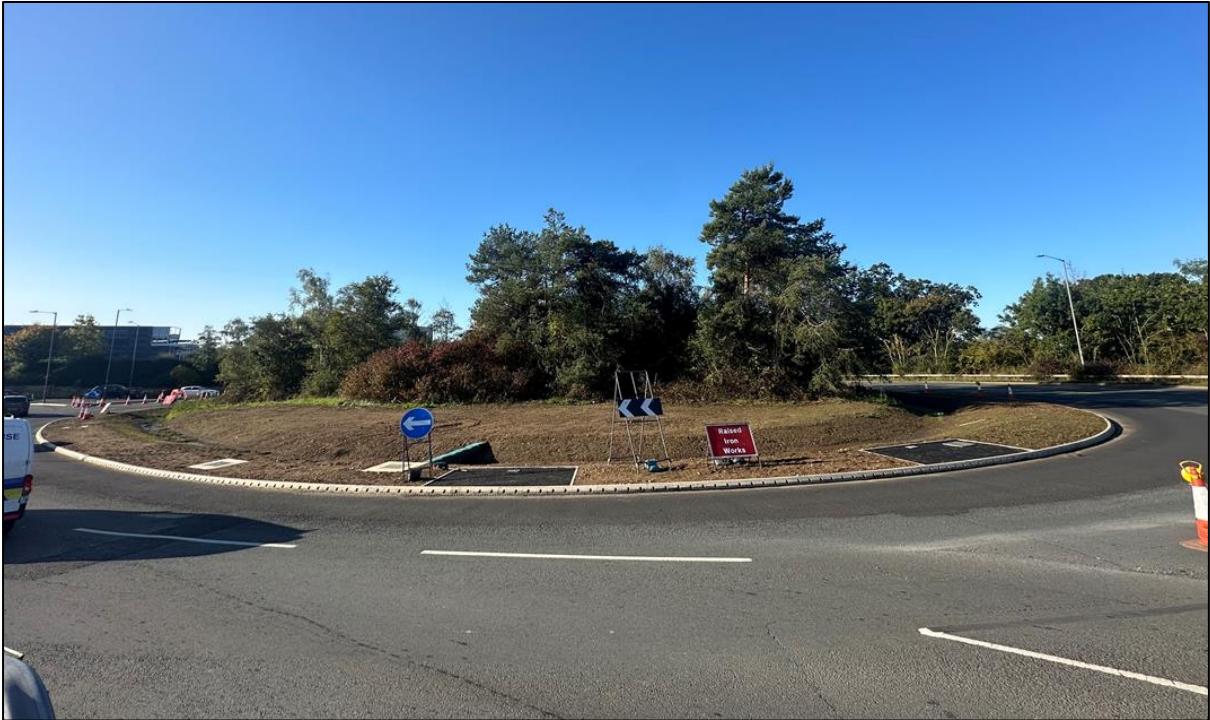
Figure 2 Queensway Roundabout – Topsoil Completion
