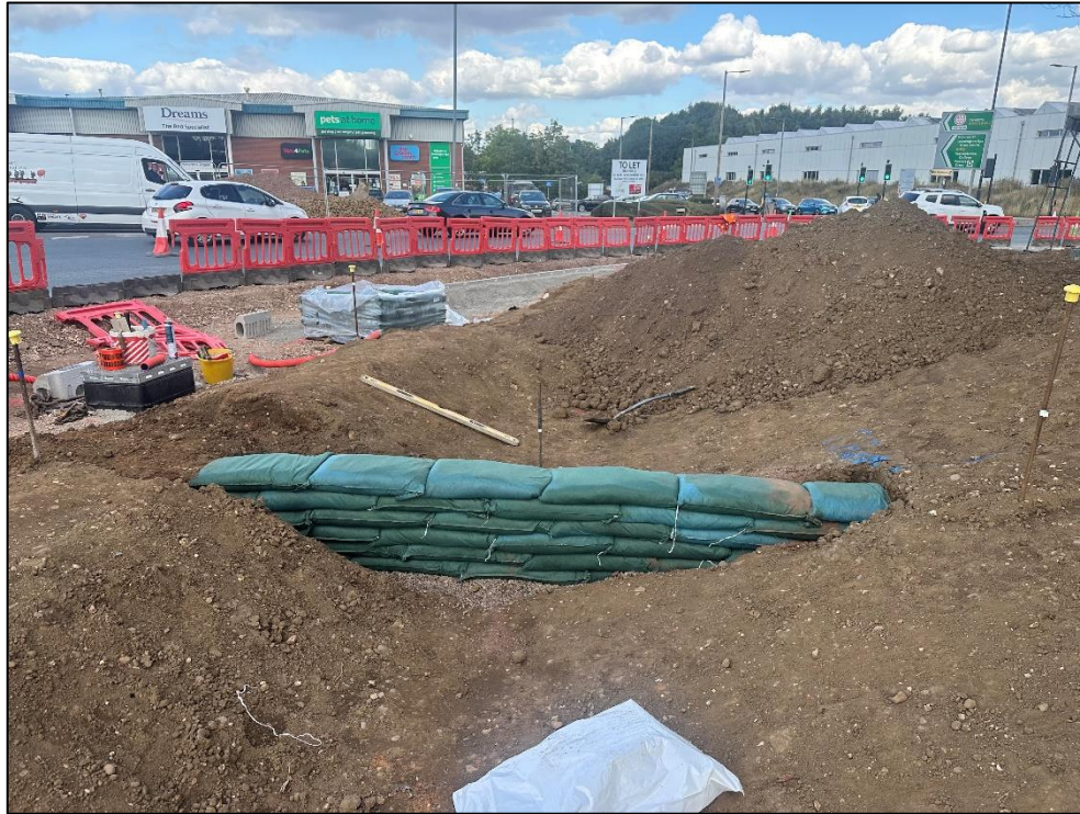
Figure 4 Old Warwick Road Roundabout – Check Dam Installation
