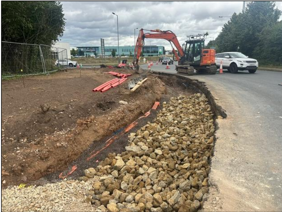
Figure 4 Old Warwick Road Roundabout– Lower Subbase and Duct Protection Installation
