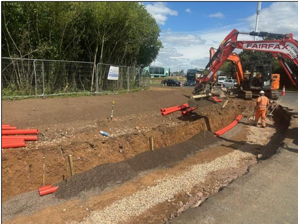
Figure 3 Old Warwick Road Roundabout - Road Box and Traffic Signal Ducting Installation
