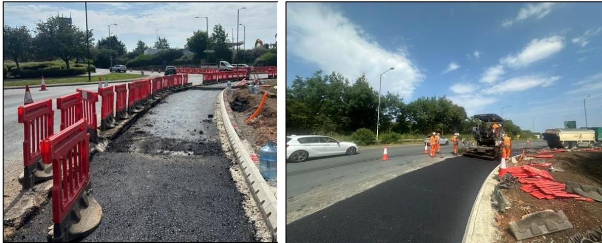
Figure 1 Phase A - Upper Road base and binder laying for the new widened carriageway lanes
