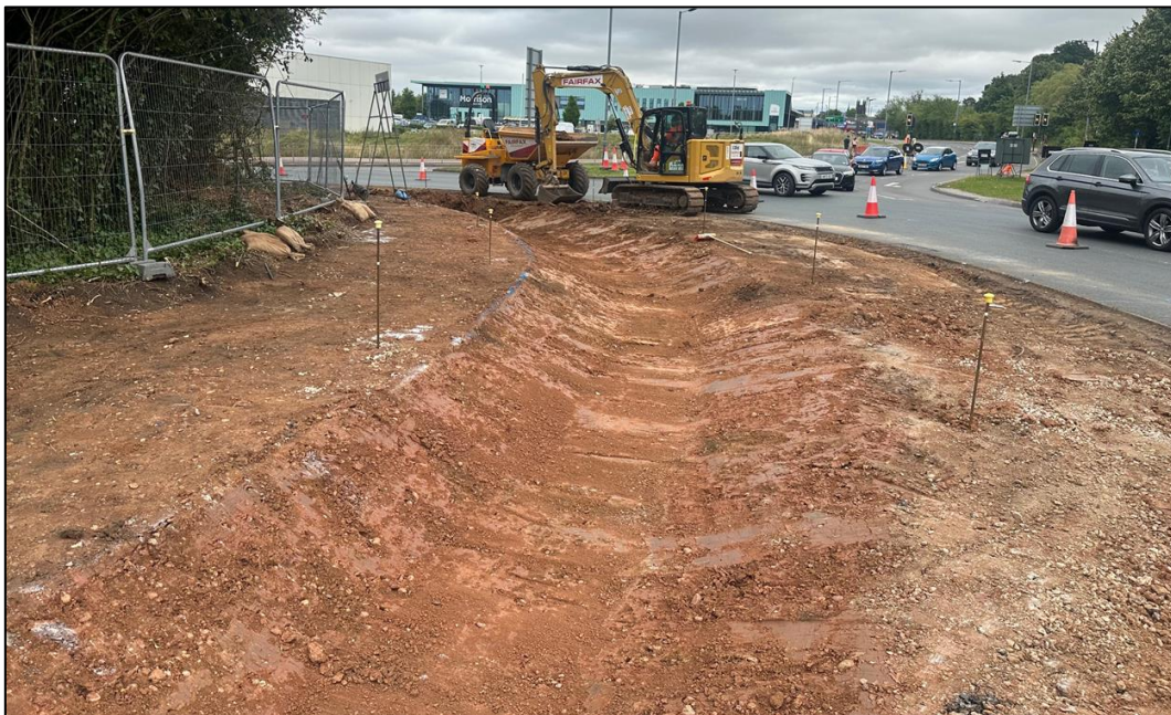
Figure 4 Old Warwick Road Roundabout Swale Construction
