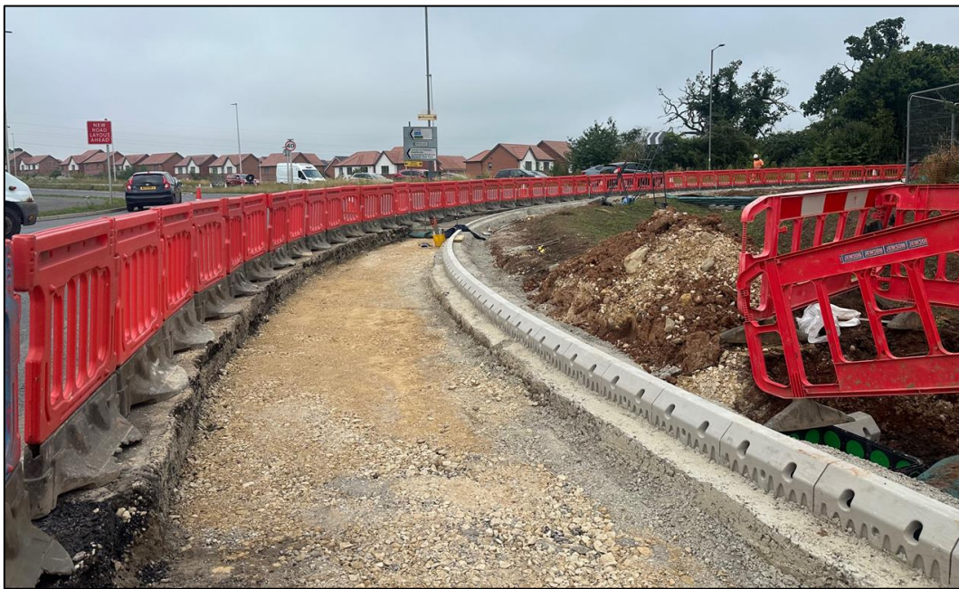
Figure 3 Queensway Roundabout – New Combined Kerb Drainage
