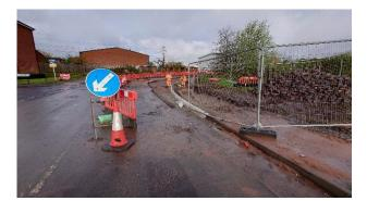
Bermuda Road / Rider Close Junction Widening works along Bermuda Road at the junction with Rider Close have continued. Traffic management was installed along the northern side of Bermuda Road opposite the junction with Rider Close to enable drainage and roadway works to be undertaken between Rider Close and Hazel Way.
