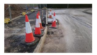
**Gulley Works by Knights Road** Due to standing water near The Bridleway and Knights Road junction the contractor installed new road gulley to minimise the risk to road users during cold weather.
