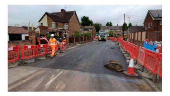
Heath End Road and Tenlons Road Junction Tenlons Road has been re-constructed up to base course and will be opened to traffic at the end of June 2023. These works were hindered by the numerous statutory utilities that required protecting before installation of new road construction could commence.
