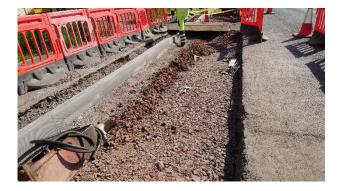
Heath End Road and Tenlons Road Junction Excavation of existing carriageway in Heath End Road is underway exposing any shallow utilities which will need to be protected to enable the road to be widened as necessary at the junction with Tenlons Road which in turn connects onto Bermuda Road and then onto the new bridge.
