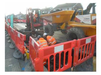
Heath End Road and Tenlons Road Junction Excavation of existing carriageway in Heath End Road is underway exposing any shallow utilities which will need to be protected to enable the road to be widened as necessary.
