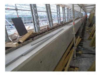
**Construction works on the Bermuda Bridge edge beam** Installation of new concrete on the northern and southern bridge edge beams is complete and timber formwork is being installed in readiness for installation of new concrete to reconstruct the edge beams to new design standards will be removed to enable new safety barriers to be installed.
