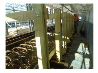
Construction works on the Bermuda Bridge edge beam Installation of new reinforcement on the northern and southern bridge edge beams is completed and timber formwork is being installed in readiness for installation of new concrete to reconstruct the edge beams to new design standards in readiness for new safety barriers to be installed.
