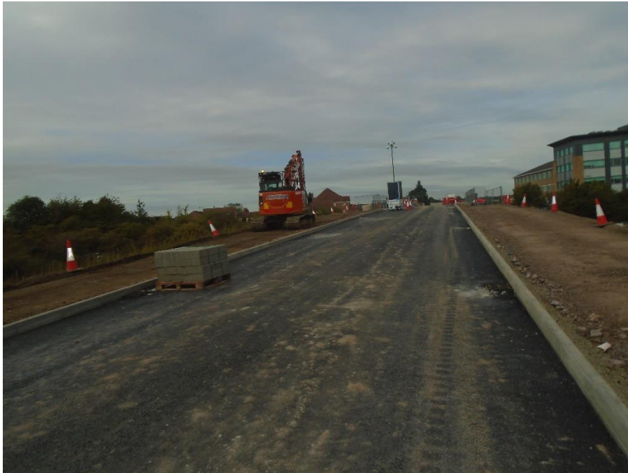
A View of the Bermuda Bridge Eastern Approach Road pavement works
