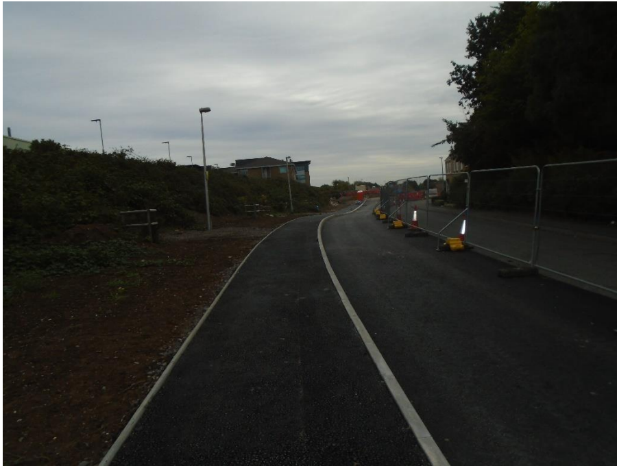
New footway along northside of The Bridleway Junction with Bermuda Road
