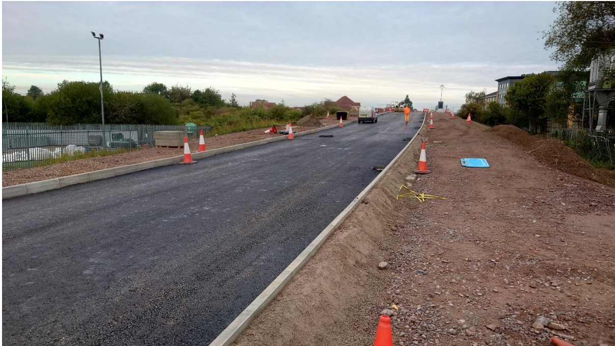
A View of the Bermuda Bridge Eastern Approach Road pavement works
