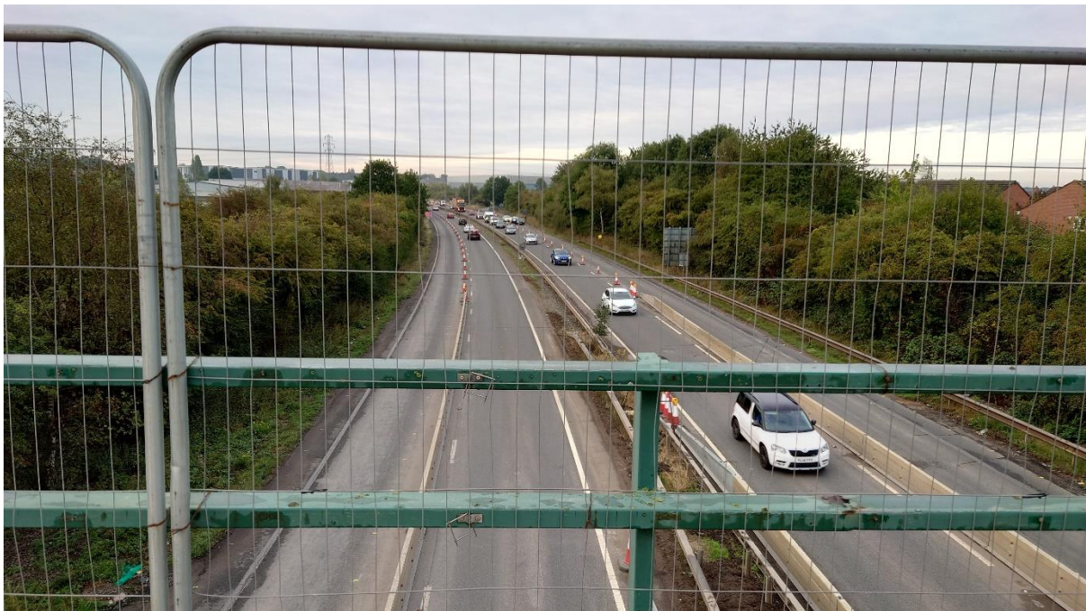
A444 looking south from Bermuda Bridge
