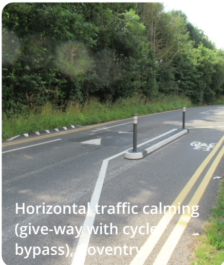
Horizontal traffic calming (give-way with cycle bypasses), Baginton
