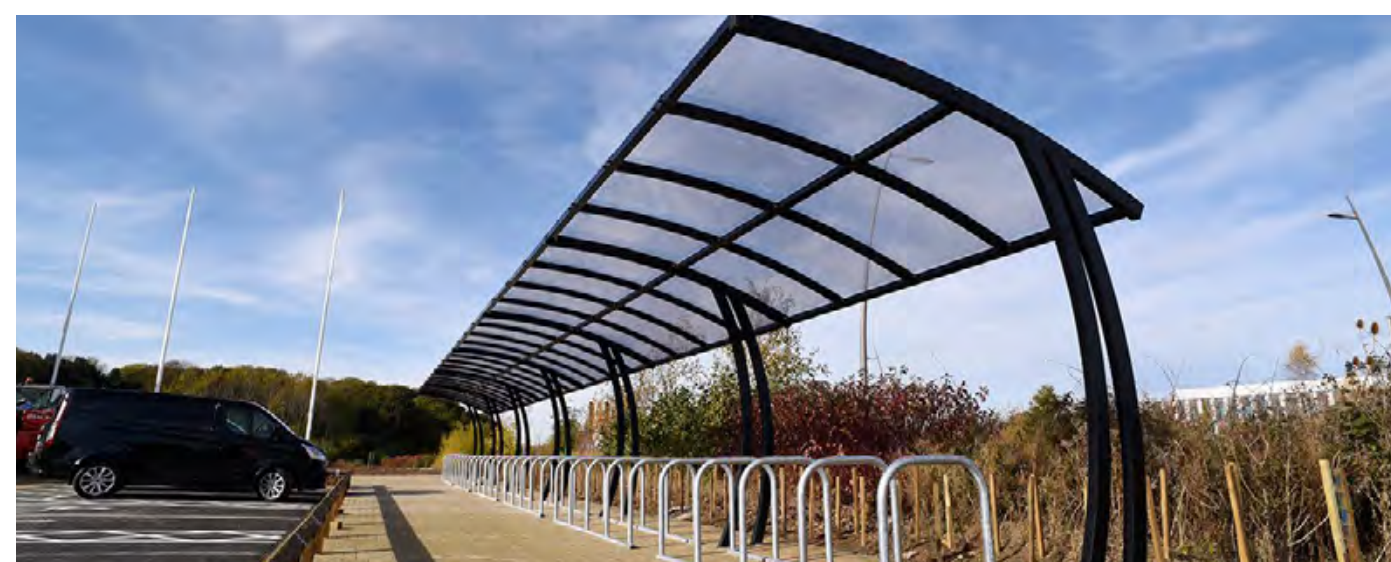
Examples of open sided cycle shelters. They require less space and could be located in tighter spots, however they are open sided and are not visually attractive when full of bikes. They do not offer the same level of security but could be accessed quicker. This type is proposed in option 3 to the west of the station entrance.
