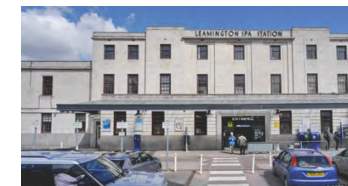
3. High volume of traffic in the forecourt area.
