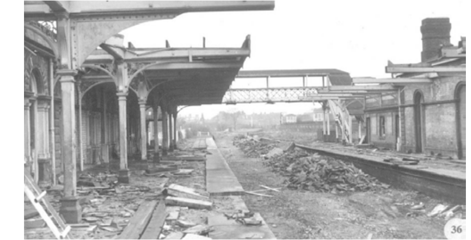
Demolition of Avenue Road Station, Leamington Spa. 1968
