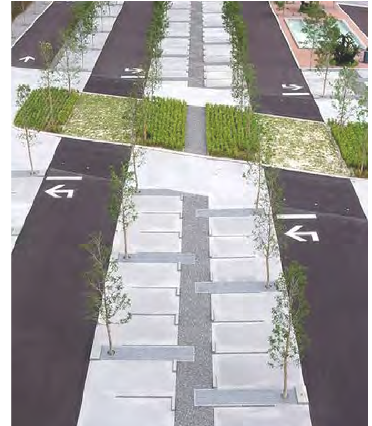
A mix of materials within car parks helps to break up the dominance of black top, adds interest and naturally segregates various spaces, without the necessity of line marking.
