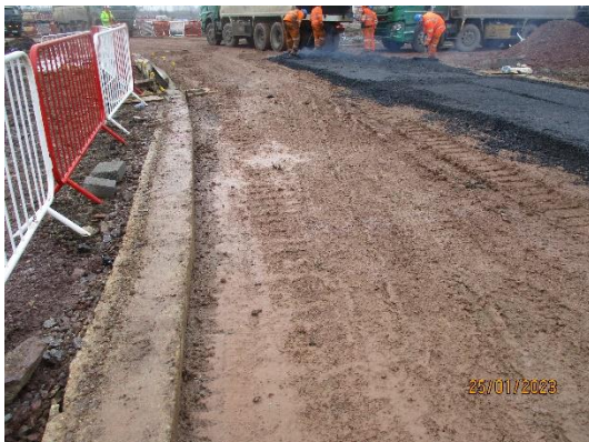
Laying Bitmac on slurry sub-base
