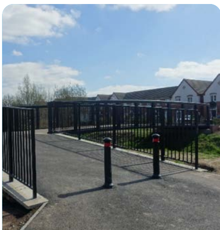
Foot and cycle bridge over Gog Brook, Warwick
