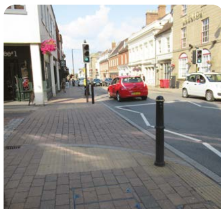
Continuous footway across side road, Warwick
