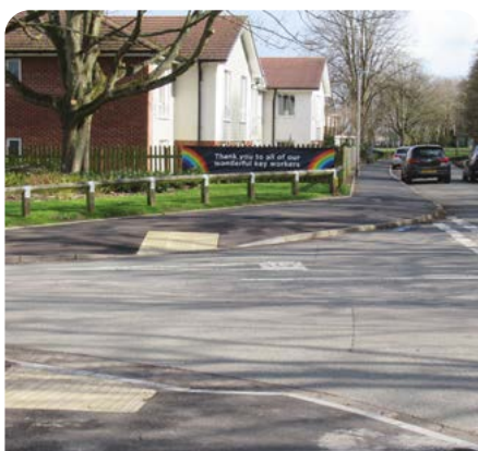
Resurfaced footway with tactile paving, Atherstone
