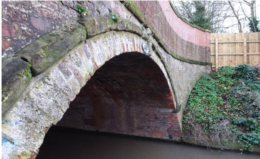
Structure B – as seen from the west
