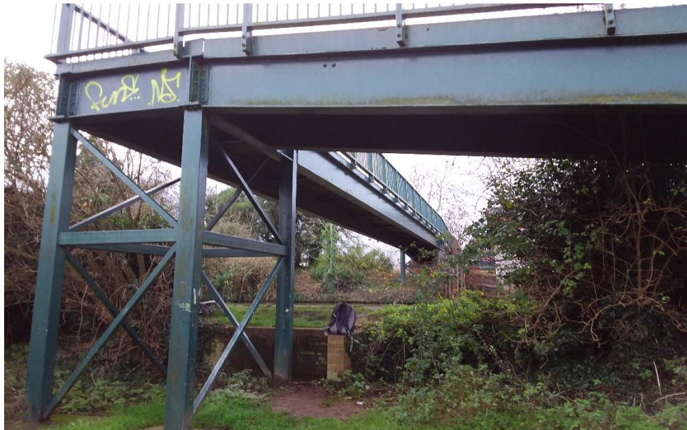
Structure A – footbridge crossing the Grand Union Canal
