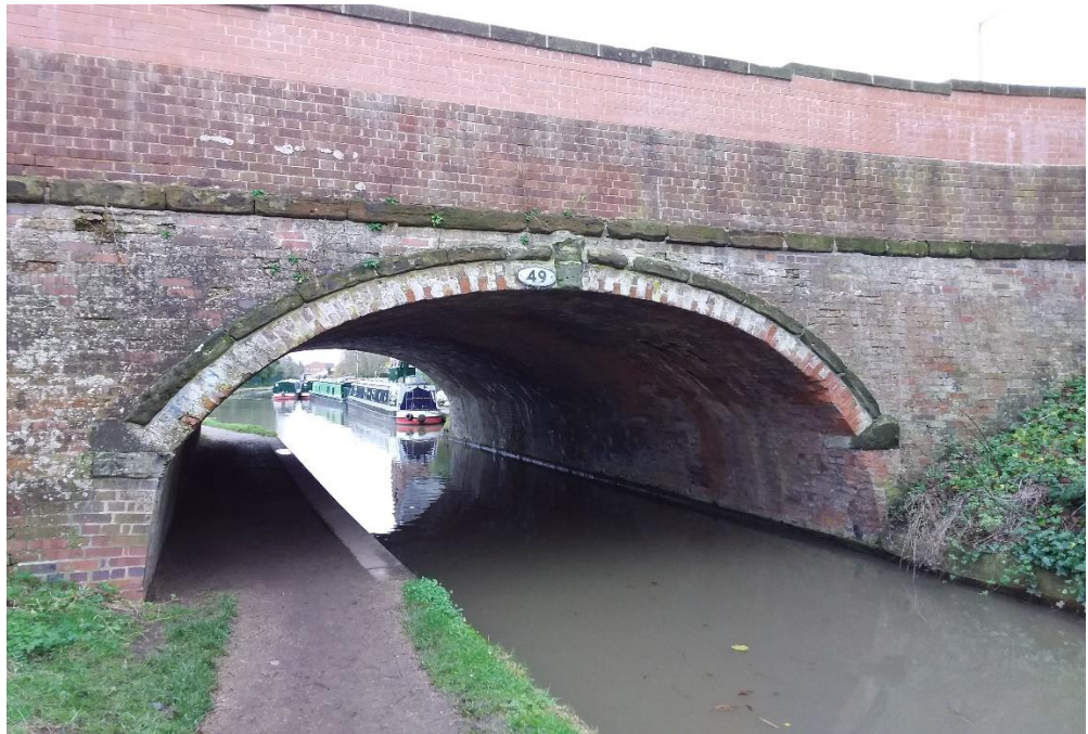
Structure B – as seen from the west
