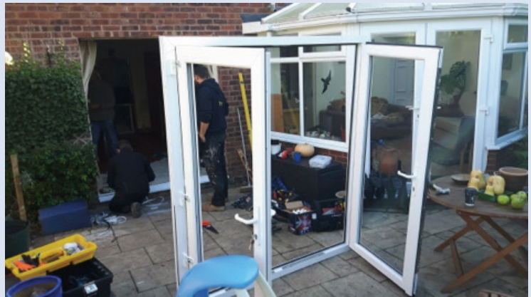
A flood proof door being installed at one property in Eathorpe.
